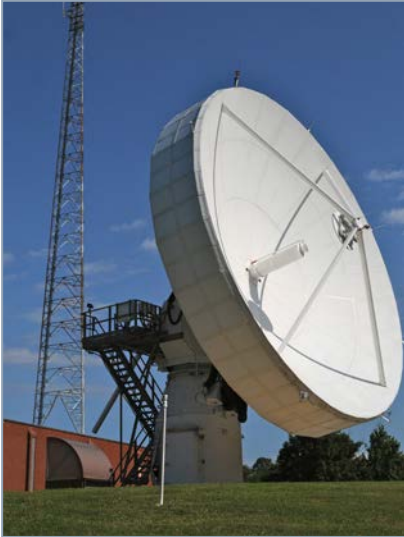
Photo of Fixed 12.2-meter Modernization of Enterprise Terminals (MET) antenna reflector assembly at Fort Belvoir, Va.
