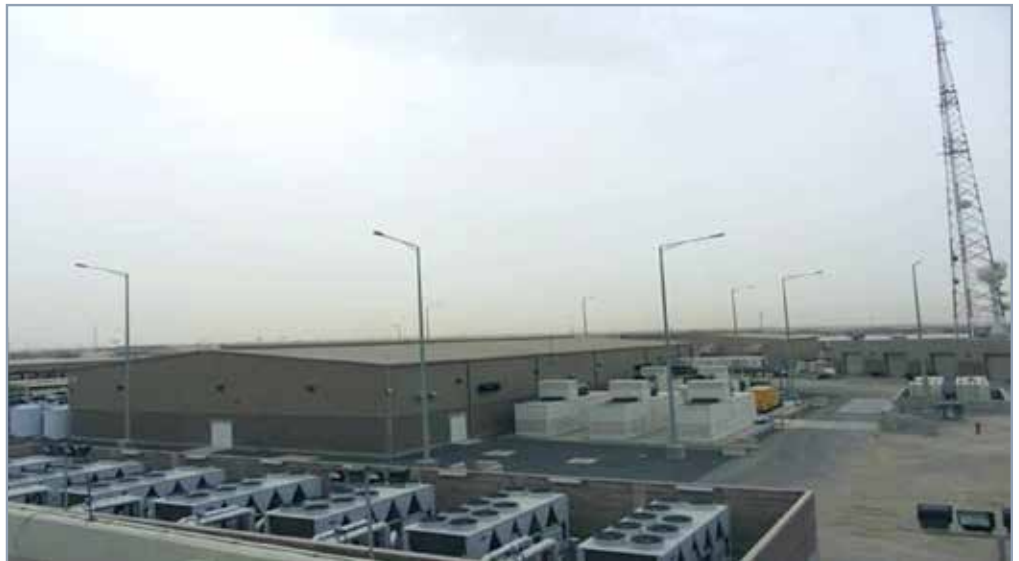
Main Communications Facility, Camp Arifjan, Kuwait.
