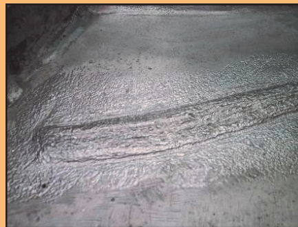
Localized crack repair treated with UIT.
