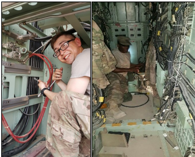
(Left) Specialist Kendrick Reed, a Radio and Communications Security (COMSEC) Repairer (94E), is replacing an Azimuth Drive Motor Cable. (Right) Private First Class Bradly Eldred, a Computer/Detection Systems Repairer (94F), is replacing High Voltage Power Cables.
