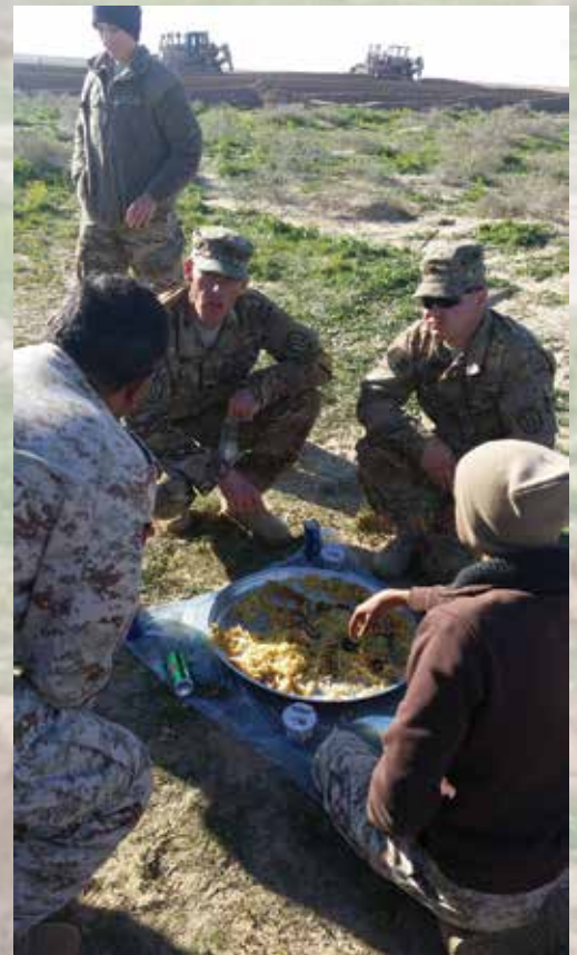
Soldiers with Utah’s 116th Engineer Company enjoy a traditional Kuwaiti meal prepared by Kuwaiti engineer forces while building an anti-tank ditch in Kuwait.
