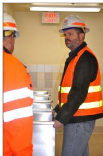
Ken Weaver (right), project manager, and an unidentified man inspect the mud room in new barracks at JB Lewis-McChord. Photos by Andrea Takash
