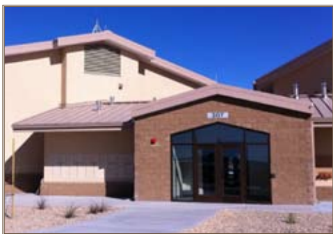
Fort Irwin's new two-story, 32,000-square-foot unaccompanied barracks features a glass entrance. Photos by Brian Clark
