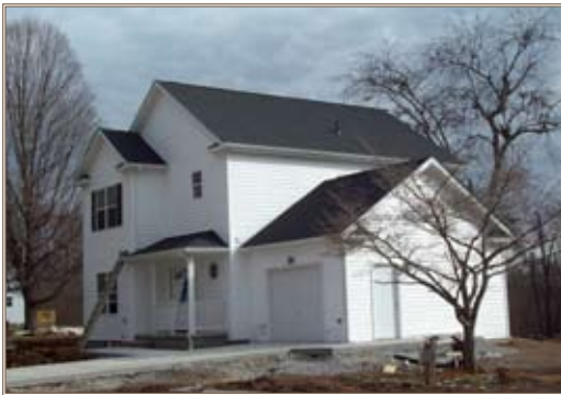
This premanufactured company grade officer house at Radford Army Ammunition Plant, Va., meets LEED Silver requirements and is built to match the traditional style of nearby residences.
