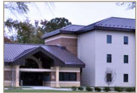
Valuable information for improving standard designs is gathered from end-state technical reviews at projects like this Joint Base Langley-Eustis Va., barracks. Photo by Dwain Scott, Fort Worth District
