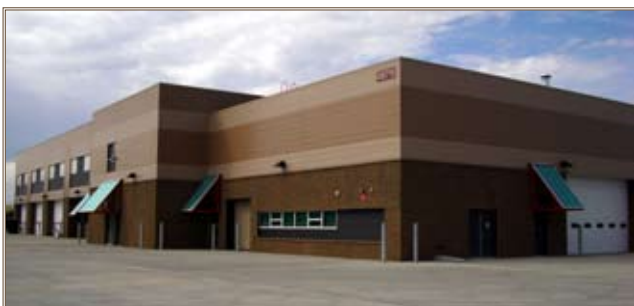
A study recommends that alignment of criteria for installation buildings, such as tactical equipment maintenance facilities like this one at Fort Richardson, Alaska, with the ISR-I would provide more accurate information for decision making. Photo by Ravin Horwell, Combat Readiness Support Team, U.S. Army Corps of Engineers
