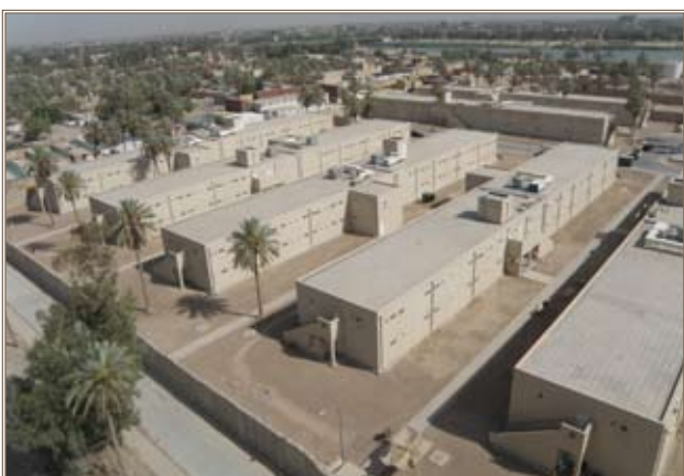
The U.S. Embassy's East End Housing Complex project in Baghdad is nearing completion. Photo by Robert Dowd
