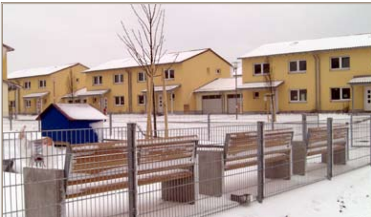
The $52 million Urtas townhouses construction project comprises 106 houses, including 22 PassivHaus units, new roads and sidewalks, utilities, playgrounds, two basketball courts, trees, landscaping and a water plant. Photo by James McPeak
