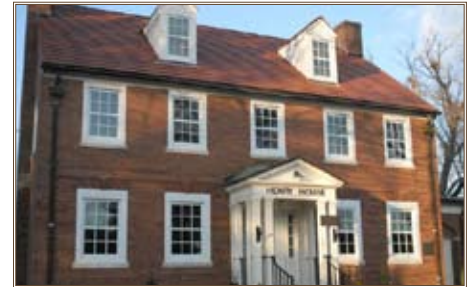
Henry House’s smart windows reduce light and heat entering the house to conserve air conditioning or let in more light to augment heating. Photo by Maureen Rose
