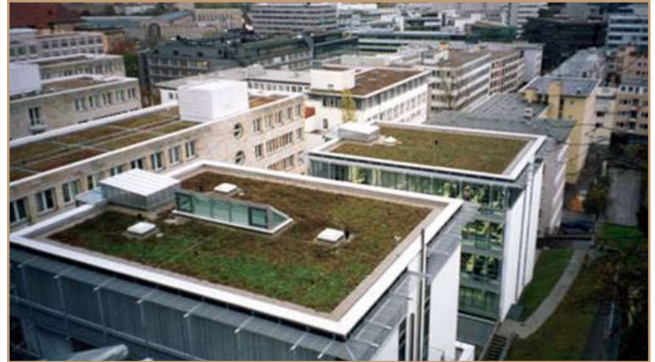
The "green roof" concept uses vegetation to help manage stormwater. Photo courtesy of Cabill, Inc. Used with permission.
