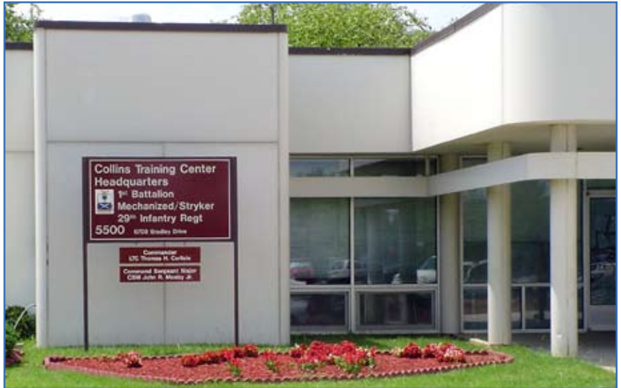
Refurbished building sign at Fort Benning, Ga., now includes the street address. Photo by Kirk Ticknor.
