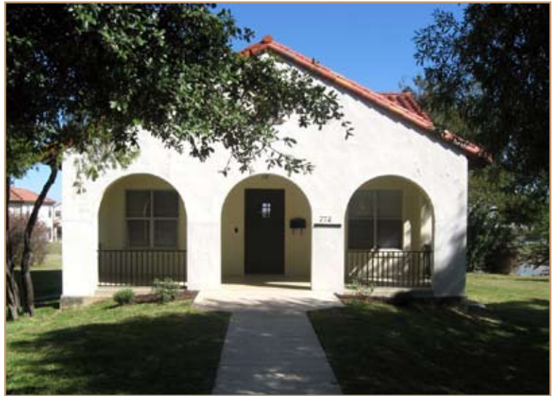
The entrance to this revamped Patch Chaffee home is wheelchair accessible. Photos courtesy of Lincoln Military Housing
