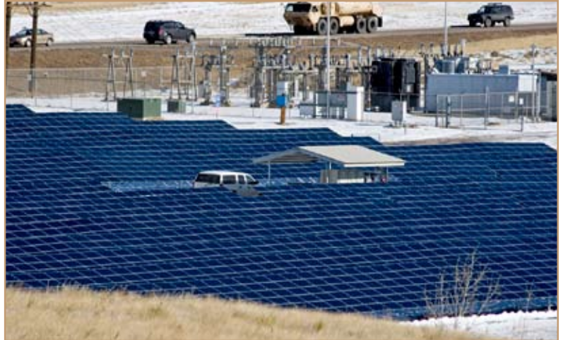
The 12-acre, 2-megawatt solar array on Fort Carson can generate enough power annually for 540 Fort Carson homes. Photo by Michael J. Pach
