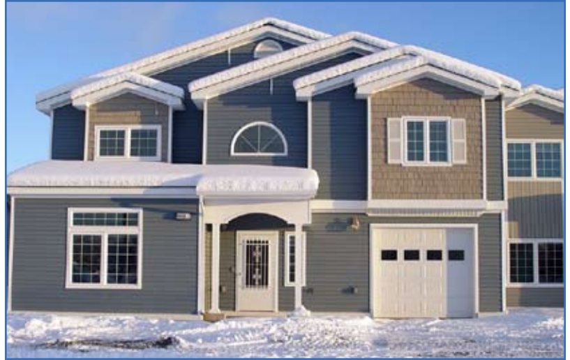
This snow-covered house is one of 67 JNCO units built in the Southern Cross community at Fort Wainwright, Alaska. Photos courtesy of USACE, Alaska District
