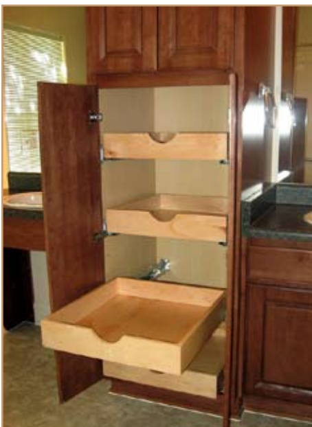
The converted bathrooms in the Patch Chaffee homes feature accessible vanities and storage units.
