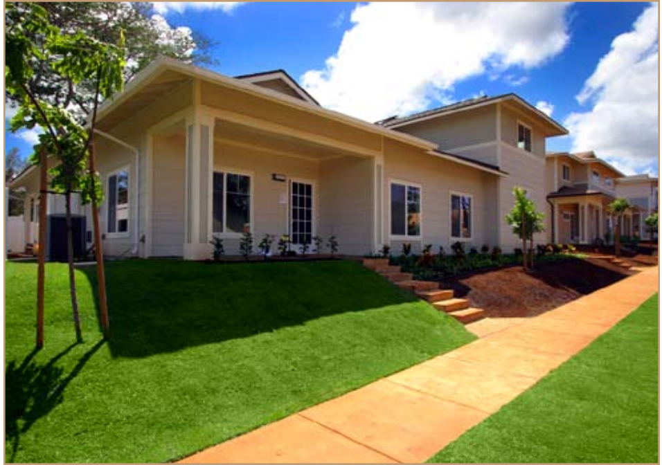
This RCI housing was built at Schofield Barracks, Hawaii, on the former Kalakaua Golf Course. Photo courtesy of Installation Management Command, Pacific Region
