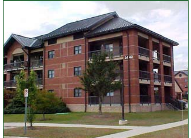
These barracks at Fort Jackson, S.C., are one example of Army permanent party barracks constructed in recent years. Photos courtesy of the Housing Division, OACSIM
