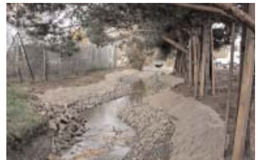
Local rocks and stones are put along the banks, while local vegetation is also being planted to help keep the banks from eroding into the stream and conserving the water's viability.
