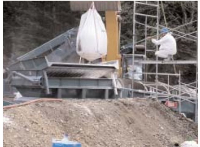
The treatment setup where the Enviroblend was added.
