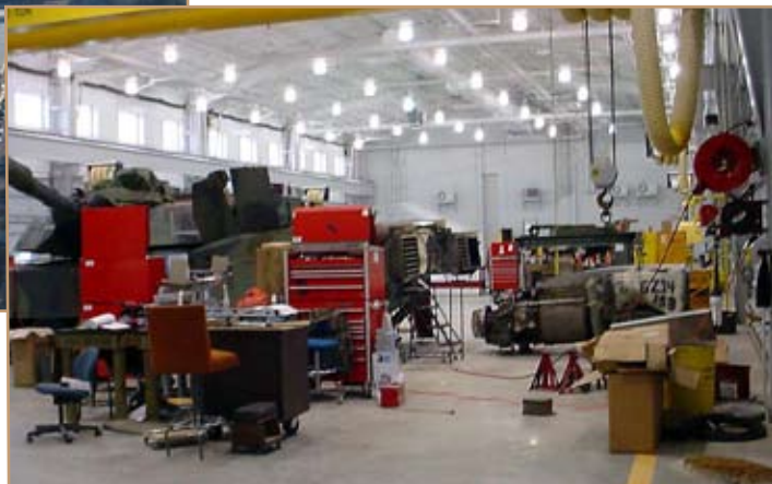
New expanded MATES Facility – no interior columns; added work space. (Photos by Kevin D. Arthur)
