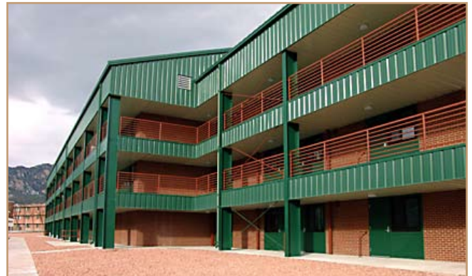
Before and after photos of the rolling pin barracks renovation project. Photos taken by Larry Lakin, Fort Carson Directorate of Public Works
