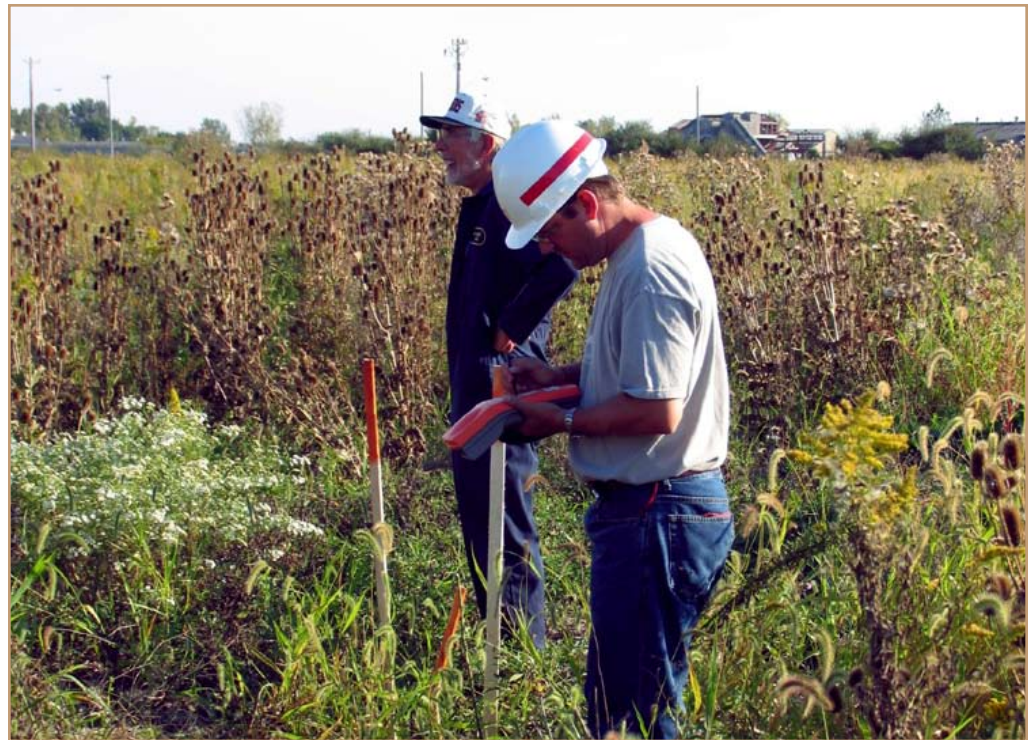
A handheld field data collection device was an efficient way to log findings as the team mapped the sewer system at JOAAP.
