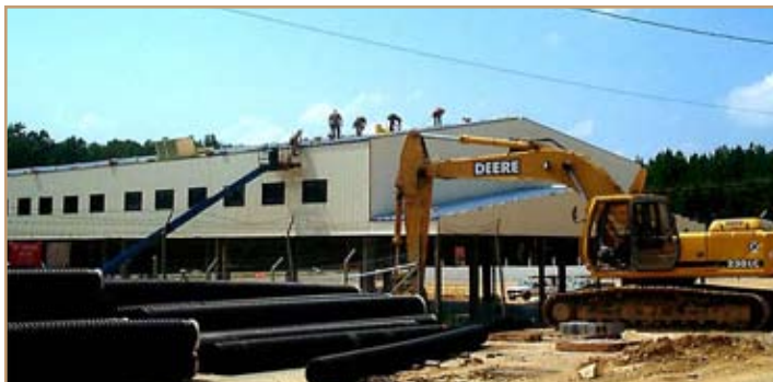
Summer 2004 construction work on expanded MATES Facility. (Photo by Jerry Rogers)
