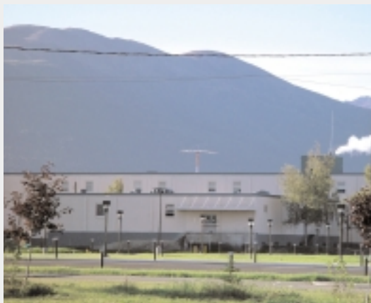
Until more new barracks can be programmed, plan B is to either renovate old hammerhead buildings to extend their lifecycles or site relocatable buildings.
