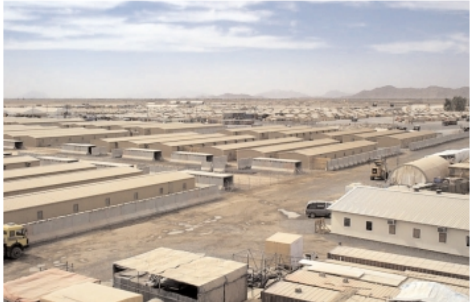
Housing constructed by USACE for Kandahar Air Field in general. There are 162 buildings with 7 rooms per building. Each room has its own bathroom and is designed for four personnel.
