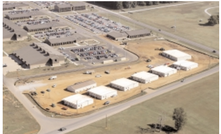
One of the Modularity sites at Fort Campbell. The Modularity buildings are the 8 new buildings in the foreground.
