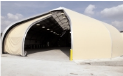
Motor pool site at Fort Stewart.
