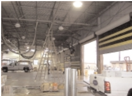
Motor Pool Super PM under construction.
