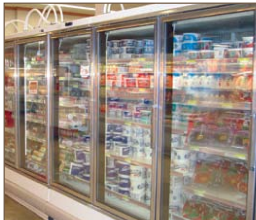
Fiber optic lighting installed in reach-in freezer display cases also reduced energy consumption. Photo by Steven Parker
