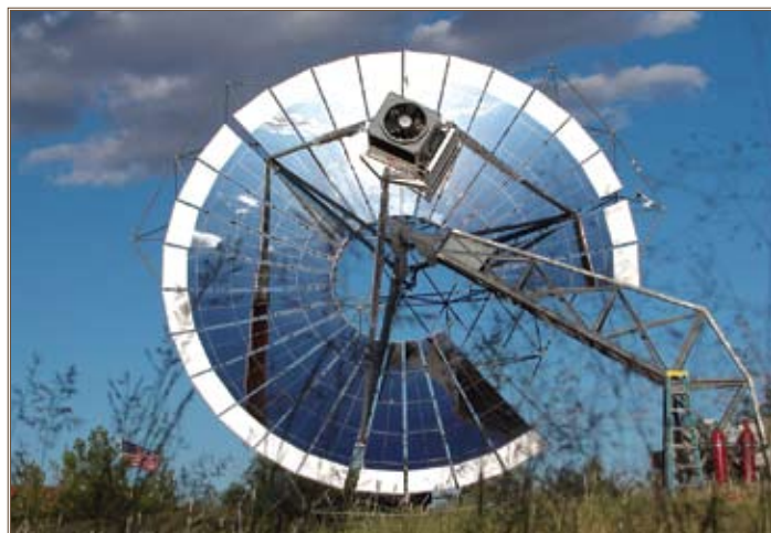
The dish/Stirling system at Fort Huachuca, Ariz., the only one in the Department of Defense, uses a parabolic dish of mirrors to focus the sun on a Stirling cycle engine coupled to a generator to produce electricity. Photo by Rich Diver, Sandia National Laboratories
