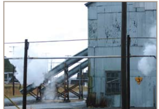
Leaking steam from distribution systems, like this one at Radford Army Ammunition Plant, Va., cause water use to rise. Photo courtesy of William Eng
