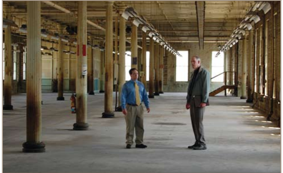
Brian Johnson (left), an electrical engineer with the EEAP, and Dave Osborn, energy manager for Rock Island Arsenal, discuss one of the 259 ECMS identified by the IMCOM-funded EEAP energy assessment. Photo by Eric Cramer, IMCOM Public Affairs Office
