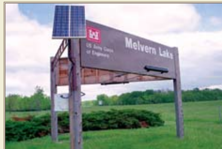
Photovoltaic panels power the light for this entrance sign to Melvern Lake, Kansas, a U.S. Army Corps of Engineers recreation area. Photo by Solar Electric Systems of Kansas City
