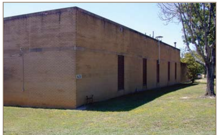
The Central Energy Plant at Fort Polk is one of the buildings that received a review of energy conservation measures by the Energy Engineering Analysis Program team from Huntsville Center. Photo courtesy of Huntsville Center
