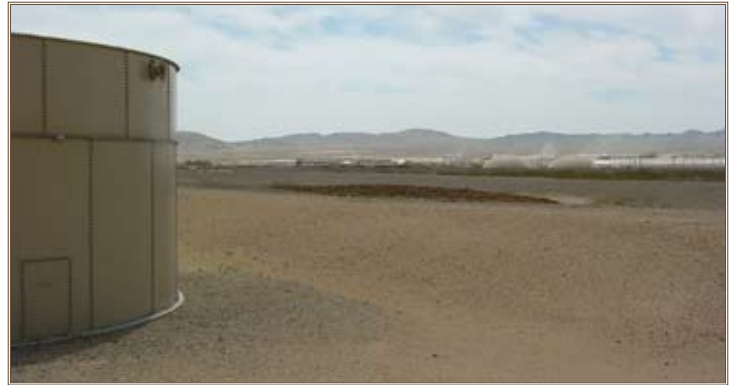
The Fort Irwin Bioremediation Landfarm is permitted to treat soils contaminated with petroleum, oils and lubricants that come from spills that occur during training exercises and from sediment removal at washracks. Photo by Justine E. Dishart
