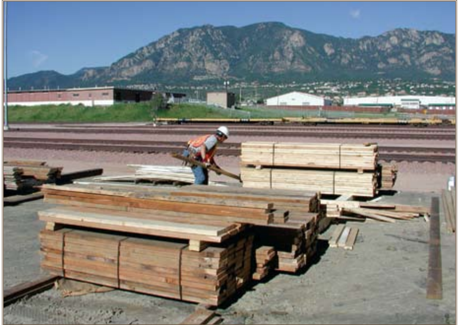
One PWTB offers guidance for recycling deconstructed building materials, like this lumber salvaged from a warehouse at Fort Carson, Colo. Photo courtesy of U.S. Army Engineer Research and Development Center
