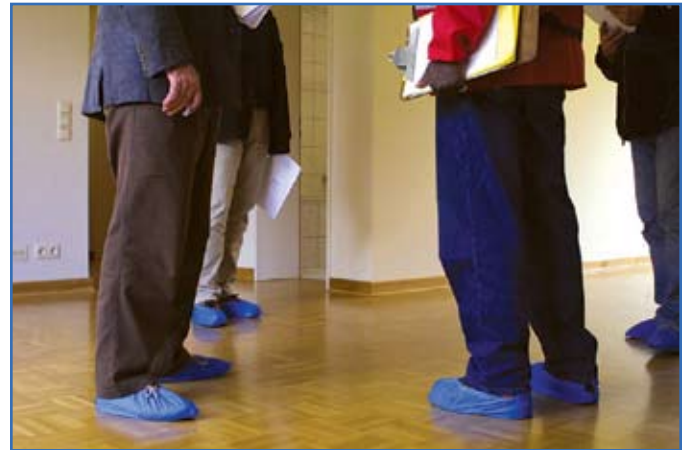
An engineering technician with the Corps' Europe District and representatives from the contractor inspect a newly renovated apartment building at Aukamm housing area in Wiesbaden, Germany. The American 110 and the European 220 outlets (on the wall in the background) make life a little easier for the families living there. Photo by Justin M. Ward
