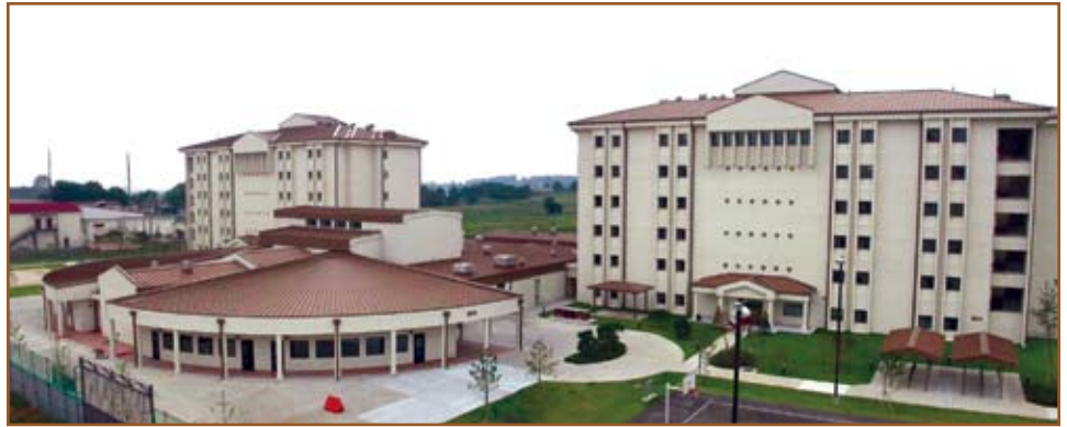
A two-building, six-story barracks combined with an 800-person dining facility at Zoeckler Station on Camp Humphreys, South Korea, is the largest of its kind in the country. U. S. Army file photo
