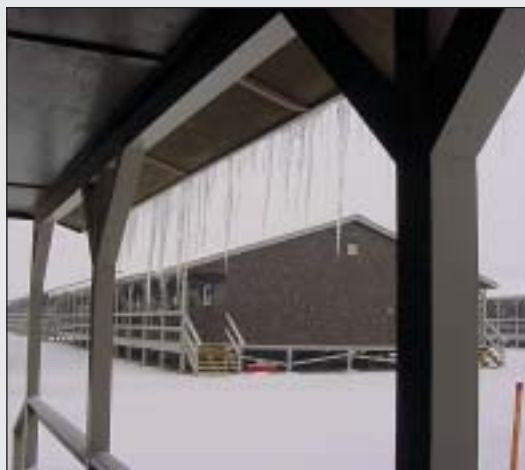
Camp Bondsteel, Kosovo in the winter. The buildings are called SEAhuts which normally have 10 living areas for civilians working in the region.
