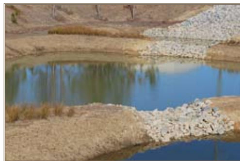
Low-impact development such as these detention ponds are the preferred method of storm-water management on Fort Bragg. Photo by Jonelle Thompson
