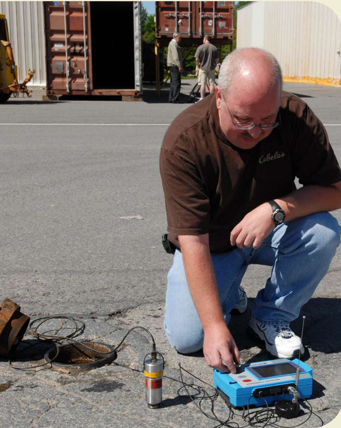
Tom Wildoner, an environmental protection specialist at Tobyhanna Army Depot, Pa., checks a drinking water leak detection sensor, part of the depot's conservation efforts that helped it win a Secretary of the Army Environment Award . U.S. Army photo. Page 14
