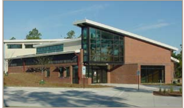
This Community Emergency Service Station at Fort Bragg will satisfy LEED Platinum criteria and save 35 percent more energy than a similar fire station built to code. Photo courtesy of Gary Poling, Savannah District
