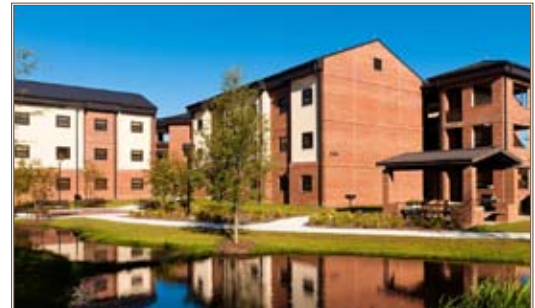
A dormitory project at Moody Air Force Base earned a Gold rating for energy efficiency and environmental sustainment from the U.S. Green Building Council. Photo courtesy of Savannah District
