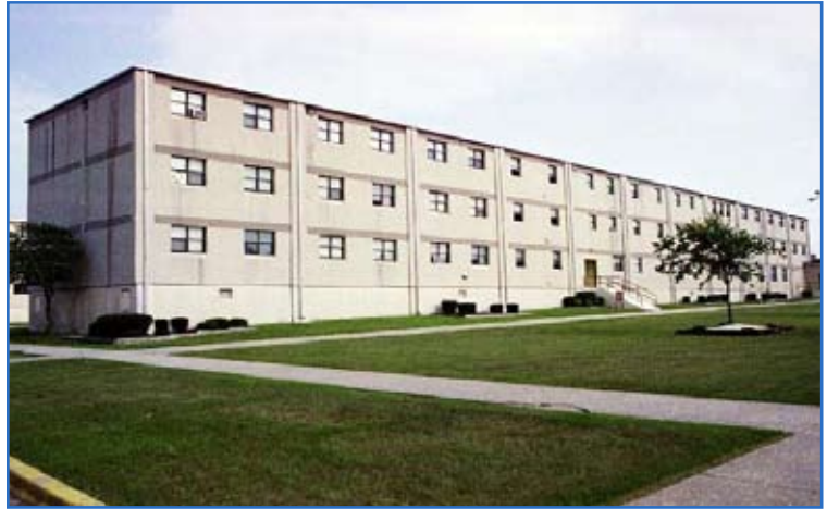
In the next 20 years, the Department of Defense will face a major compliance challenge as more than 100,000 buildings become 50 years old or older. Photo by RC Goodwin & Associates
