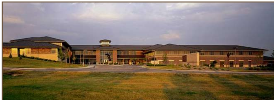
This Ellsworth Air Force Base office building is designed with narrow wings that lower energy use by reducing air conditioning, relying on cross ventilation and providing more natural light. Photo by Mark Gillem, Urban Collaborative
