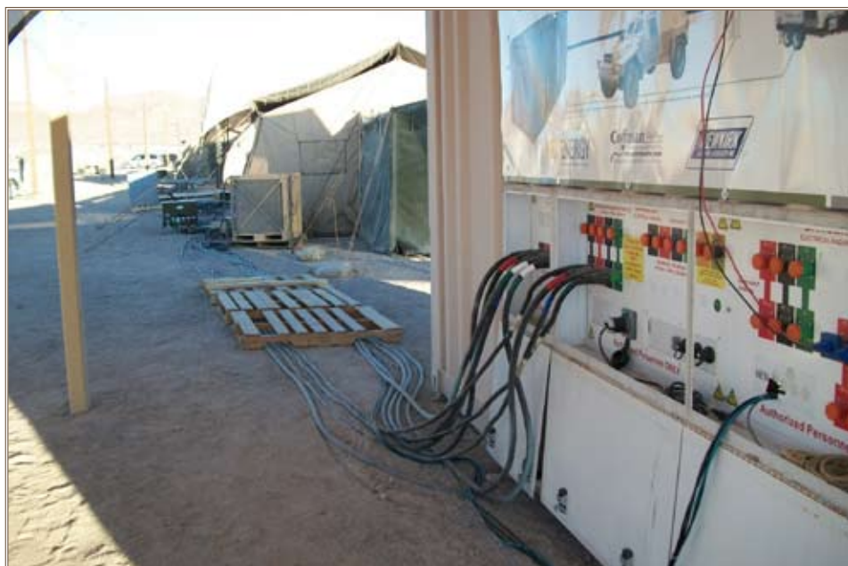
An electronic power control and conditioning module, potentially a vital part of a micro-grid, takes a variety of electrical inputs from sources as diverse as unsteady grids in foreign nations, generators and renewable energy resources, and combines this mix of spotty, inconsistent power sources into a single smooth flow of computer-grade electrical power.” Photo courtesy of U.S. Army
