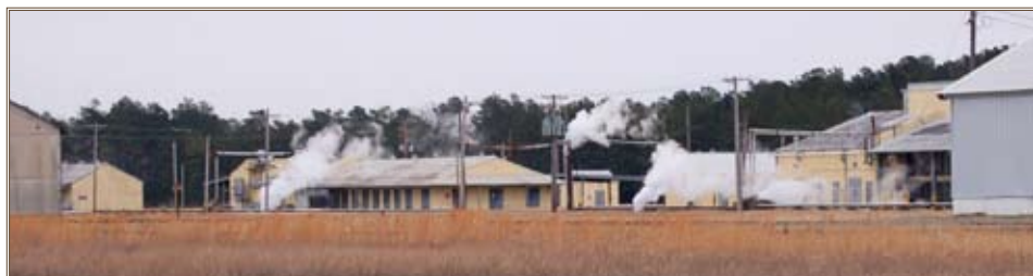
Miles of above-ground steam line at Pine Bluff Arsenal will be removed through an ARRA-funded infrastructure upgrade project. Photo by Ray Fish, Pine Bluff Arsenal
