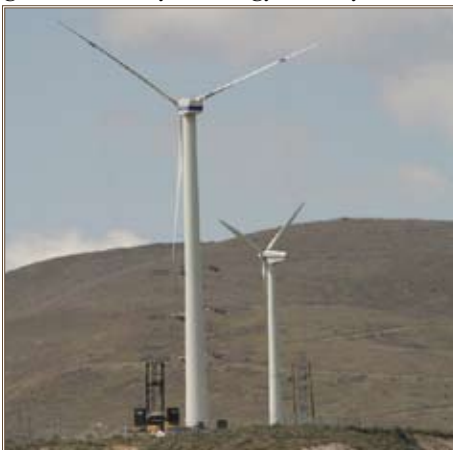
A wind turbines project at Camp Williams, Utah, will help the Army achieve renewable energy goals.
