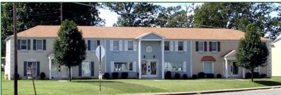
Older apartment-style housing is found in Lee Village at Fort Campbell.
