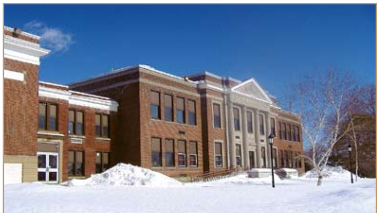
This school building was renovated by Mike Treanor and Associates into homes for Fort Drum military families.
