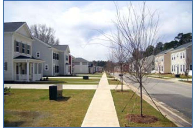
The first 56 out of 599 homes to be built in McGraw Village at Fort Benning, Ga., were delivered in March. Photo by Mickey Kropf
