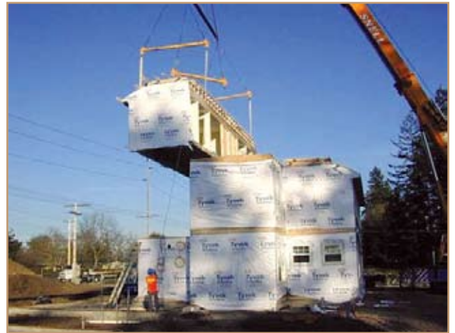
A modular home is set into place at Fort Lewis, Wash. Photo by Joyce Curtis
