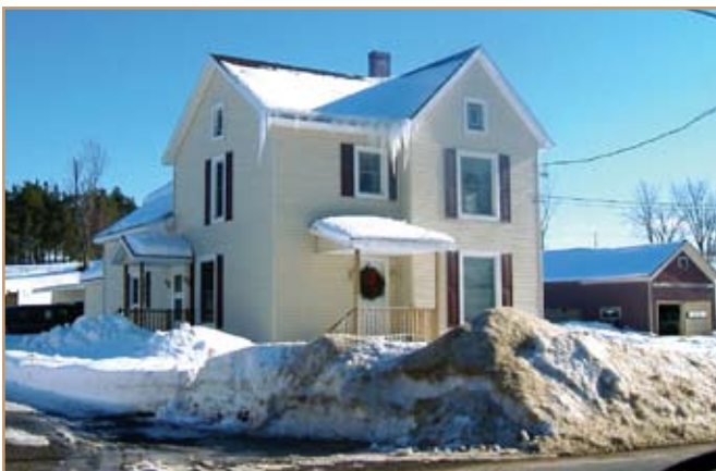
The Smith family found this home near Fort Drum through the Domestic Lease Program. Photos by Barbara Dindl, Fort Drum Housing Office
