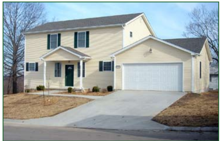
A new single-family residence rests on the old foundation.
