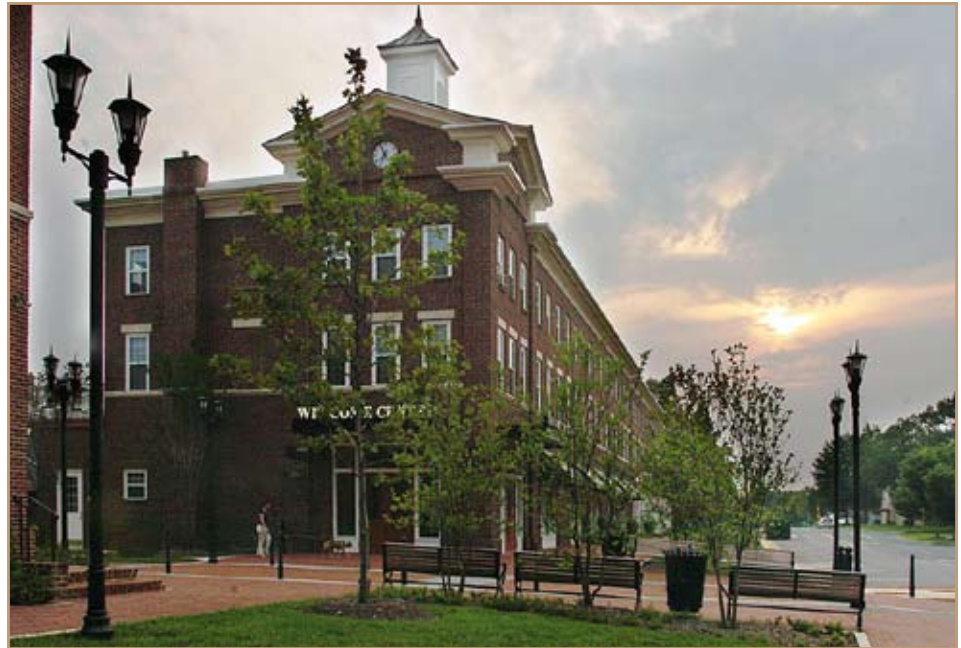
With retail shops at ground level and residential units above, Fort Belvoir's Town Center demonstrates mixed-use development. Photo by Marny Malin
