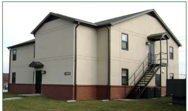
Despite an exterior identical to standard military construction, the two-story, 4,322 square-foot container building's sturdy steel frame boasts superior resistance to damage by wind, fire, mold and moisture.
