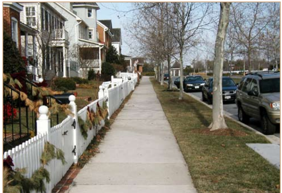
Six-foot wide sidewalks, a buffer zone of equal width and shade trees help make this community walkable. Photo by Jeff Springer
