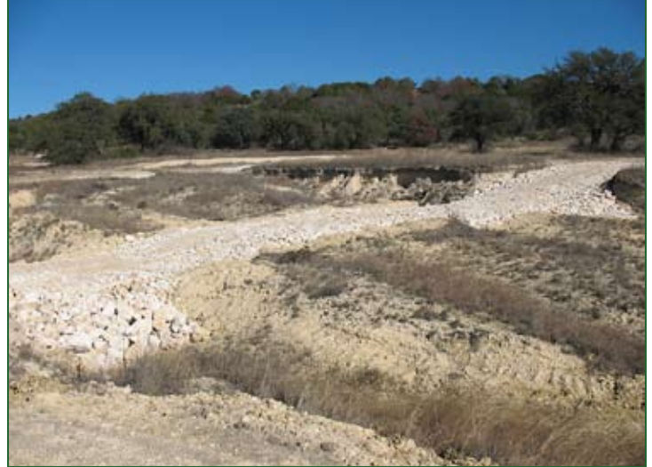
The gully plugs, which are rock structures, capture a majority of the sediment throughout the training areas and serve like bridges for tanks and other vehicles. Photo courtesy of Christine Luciano
