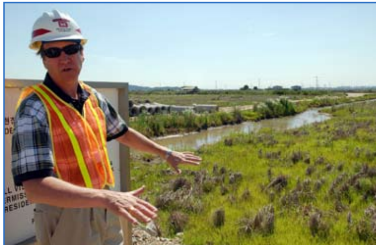
Fred Davis Jr., with the Korea Relocation Program Office of the Army Relocation Branch for the U.S. Army Corps of Engineers, Far East District, shows a rice paddy that will be drained and filled for development at U.S. Army Garrison Humphreys, South Korea. All top soil and growth must be removed before fill dirt can be placed. Photos by Fred W. Baker III
