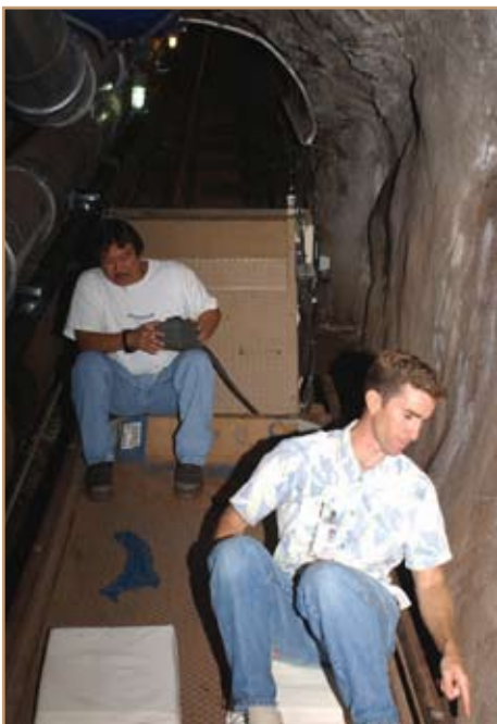
Wayde Nakai (left), water plant supervisor, and Kent Anderson, a Directorate of Public Works water system engineer, ride in a car down the tunnel that burrows about 1,200 feet at a 30-degree angle to reach the Schofield-Wheeler aquifer nearly 600 feet below ground. Photo by Jeremy S. Buddemeier
