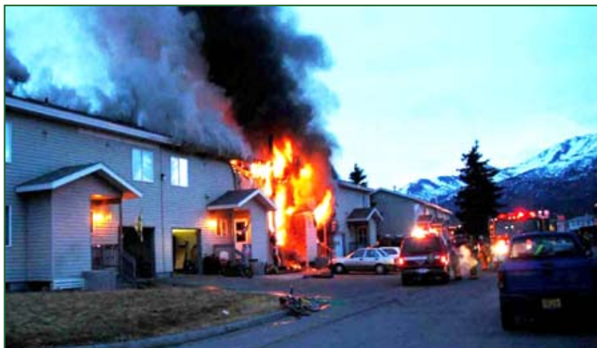
A fire rages in a family housing unit. Photo courtesy of the Office of the Assistant Chief of Staff for Installation Management
