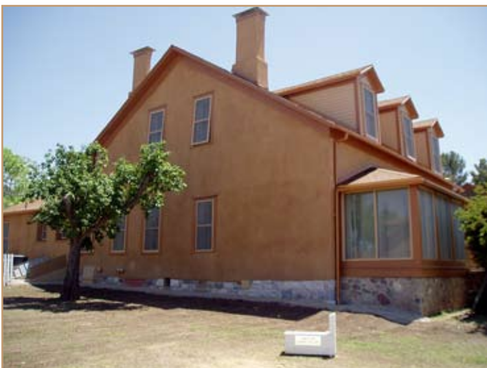
Restoration of the 1884 Miles House in Cavalry Park at Fort Huachuca, Ariz., is complete. Photo by Mike Zurcher
