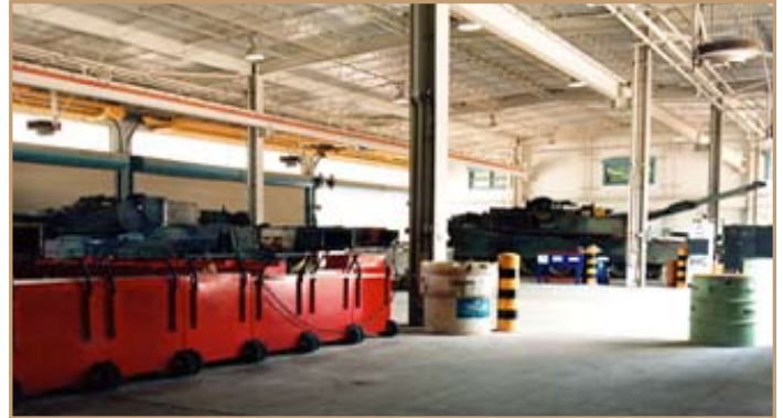
This armored vehicle maintenance facility at Fort Knox, Ky., is an example of the type of facility for which standard designs are being developed. Photo from the Installation Design Standards web site
