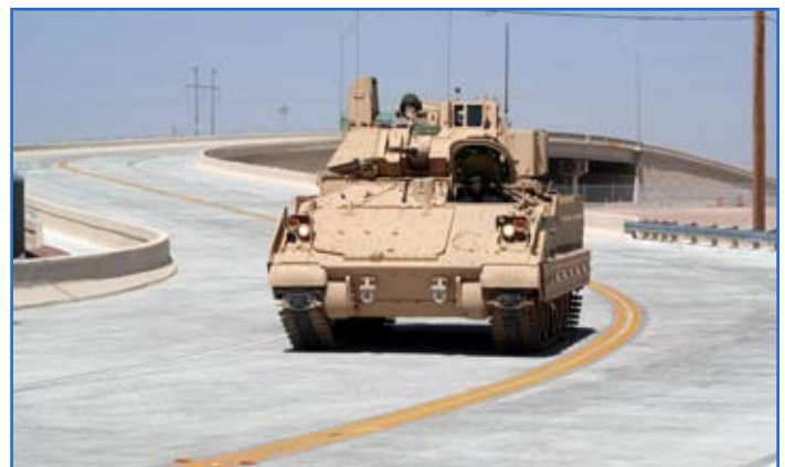
A military vehicle cruises over Haan Bridge. Although completed, the bridge won't be open to civilian traffic until adjacent road work by the Texas Department of Transportation is completed in September. Photo by Melissa House, Fort Bliss Public Affairs Office
