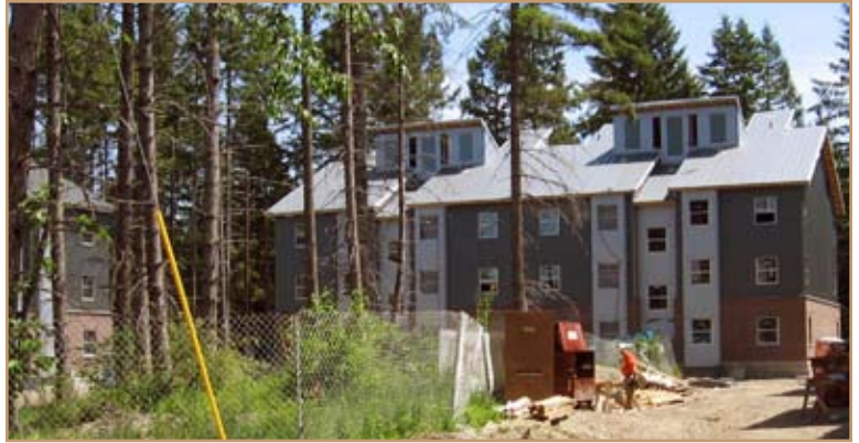
Fort Lewis's Jackson Avenue Barracks designers created four smaller buildings oriented around a courtyard of existing trees and added high windows to bring in more light and reduce electricity use. Photo by Bruce Hale
