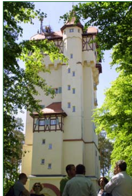
While touring the Grafenwöhr installation, high-ranking Israeli visitors gather outside the famous water tower, a half-timbered structure completed in 1910. The tour's purpose was to show the visitors the progress of the Efficient Basing-Grafenwöhr program, which builds up the installation while retaining traditional architectural styles. Photo by Justin M. Ward
