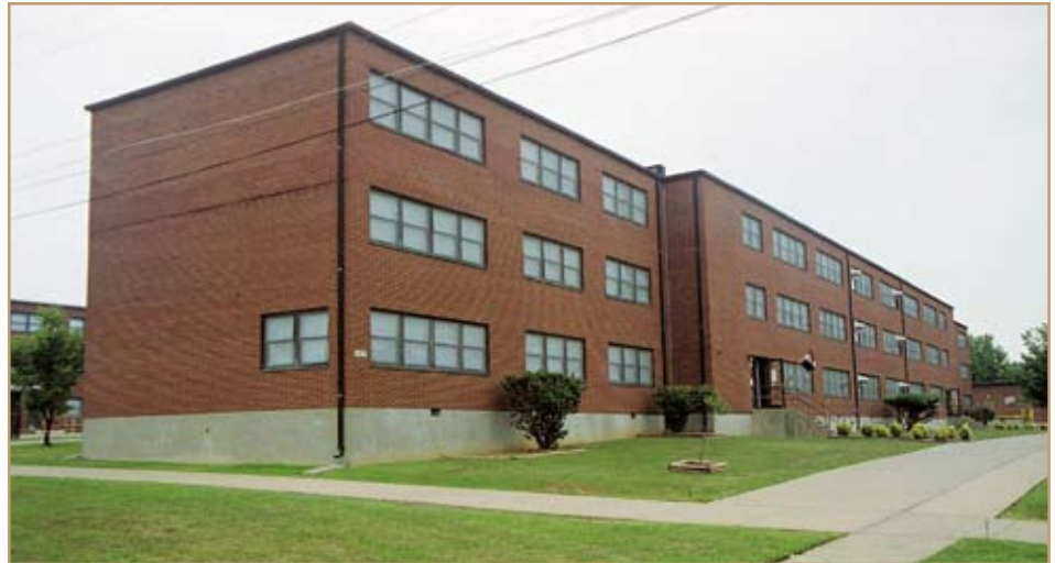
The “Rolling Pin” design of these barracks at Fort Knox, Ky., is typical of Unaccompanied Personnel Housing built during the 1960s. Photos courtesy of R.C. Goodwin and Associates
