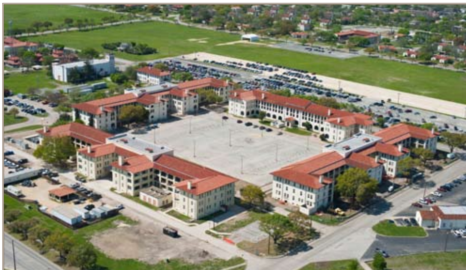
Three of the four historic buildings in this grouping are being renovated to provide additional space for IMCOM, and IMCOM's headquarters building will be constructed in the middle. The post theater (upper left) is also being renovated. Photos courtesy of U.S. Army Corps of Engineers
