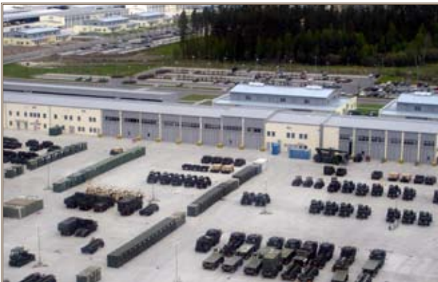
New motor pools are among the EB-G construction projects.
