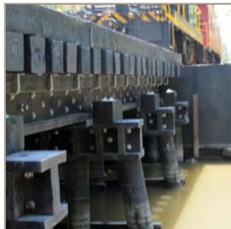
An Army Transportation School locomotive and caboose crosses a bridge constructed of RSC material. Photo by Tetaun Moffett
