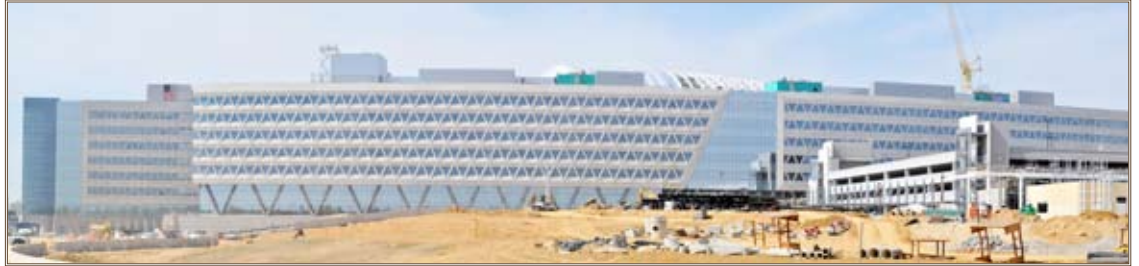
The NGA Main Office Building goes up amid BNA infrastructure construction.
