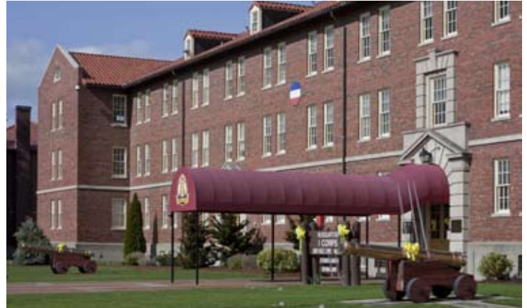
The newly renovated Building 2025 at Joint Base Lewis-McChord, Wash., stands ready for returning I Corps Soldiers. Photo by Dane Gregory Meyer, DG Studio
