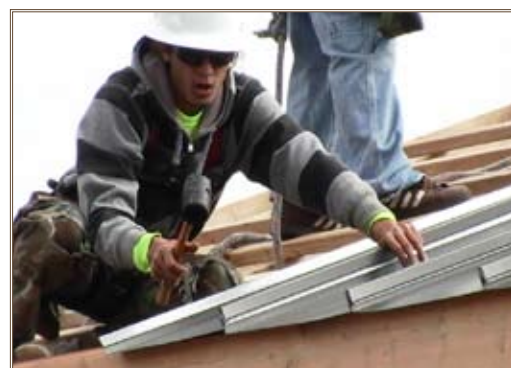
Workers then install the combined unit on the roof joists.
