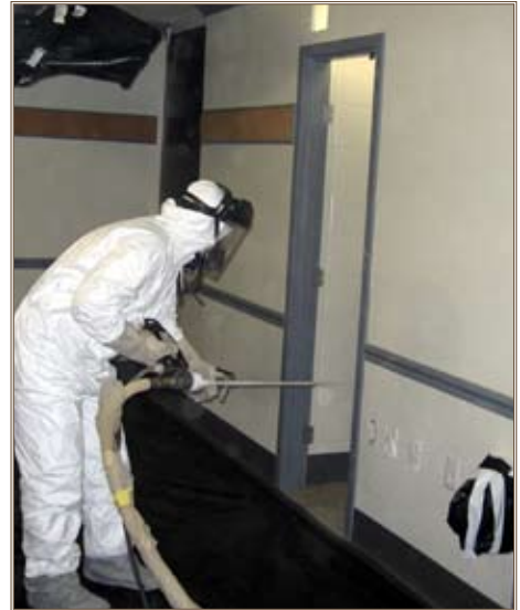
Appropriately suited, a worker blasts mold off walls using dry ice pellets as part of a mold abatement test at Fort Polk. Photo courtesy of ERDC
