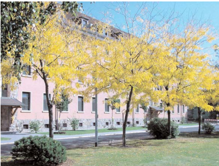
Trees planted create park-like environment for single soldier barracks at Spinelli Barracks, Mannheim. Exterior plaster, paint, window, door details and entrance canopy complement original yellow sandstone, plaster and clay tile roof architecture of 1934.
