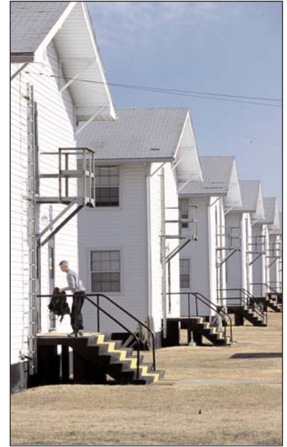
The WWII barracks are symbolic of this historic post.
