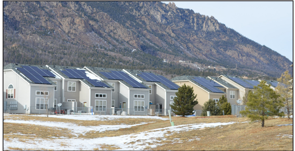
SolarCity finished installing 3 megawatts of solar systems this summer on the roofs of privatized family housing units at Fort Carson, Colorado. The solar energy from family housing units is providing 128 percent of the family housing residents' electricity. (Photo courtesy of SolarCity)
