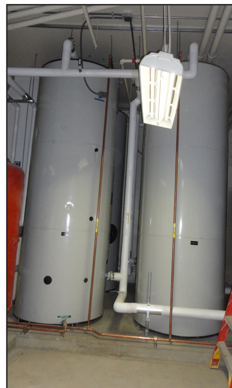
New heat pumps and storage tanks, replacing fuel oil boilers and outside equipment, are located within the newly renovated barracks at Fort Hunter Liggett, California. The Transient Training Enlisted Barracks were upgraded to create net Zero Energy Buildings. (U.S. Army photos)
