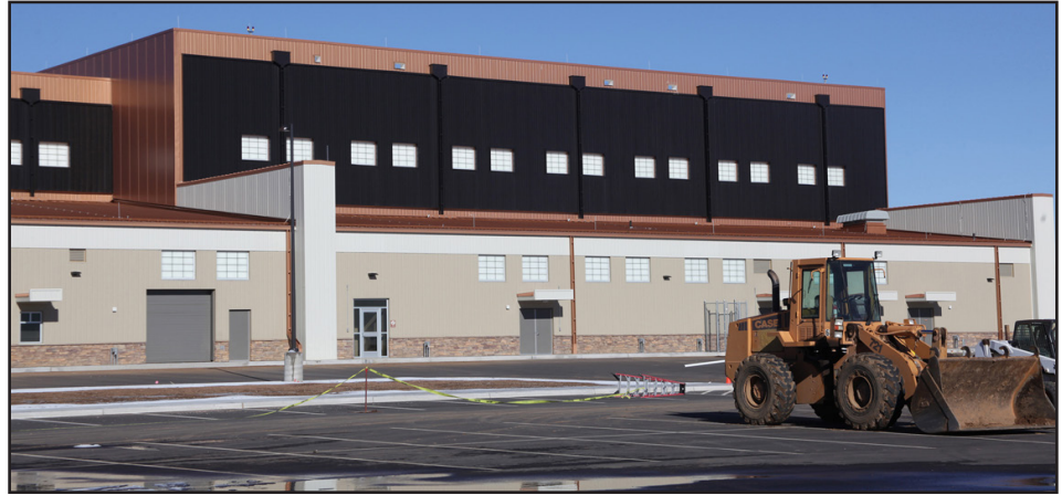
This construction photo shows the simplicity of the transpired solar walls for the 13th Combat Aviation Brigade Aviation Support Battalion Hangar at Fort Carson, Colorado. The system blends into the façade without being an eyesore. (U.S. Army photo)
