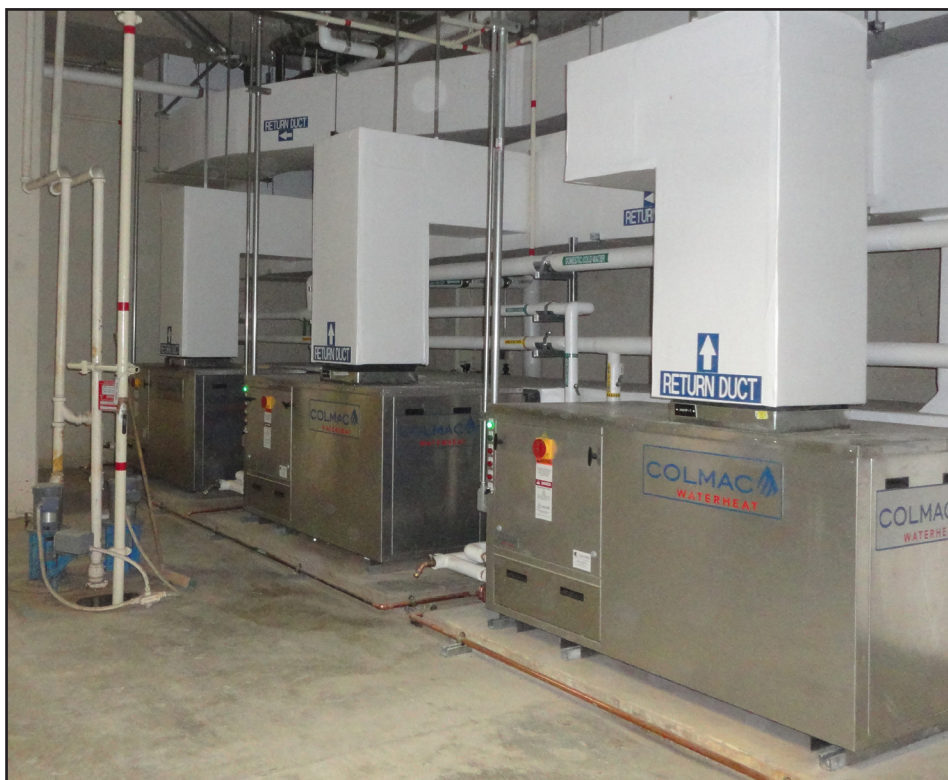
New heat pumps and storage tanks, replacing fuel oil boilers and outside equipment, are located within the newly renovated barracks at Fort Hunter Liggett, California. The Transient Training Enlisted Barracks were upgraded to create net Zero Energy Buildings. (U.S. Army photos)
