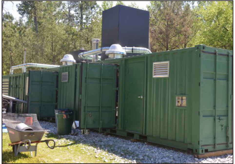
The battalion-scale Waste to Energy Conversion Green Energy Machine converts 3 tons of trash into 100 gross kilowatts of energy at Fort Benning, Georgia. (Photo by Danielle Davis)
