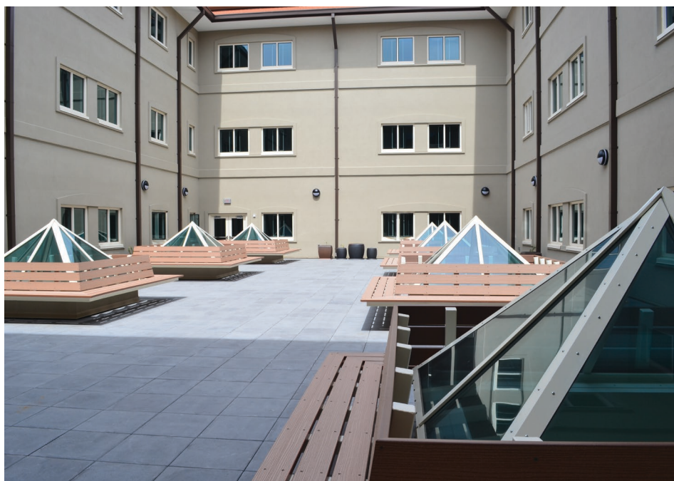
The inner courtyard of the new general instruction building for the Defense Language Institute Foreign Language Center at the Presidio of Monterey, California. The courtyard sits on the roof of the second floor which allows all interior facing rooms to receive sunlight through windows that reduce the use of interior lighting and electricity. The courtyard also features multiple skylights to provide natural lighting to the assembly hall below. All rainwater that lands on the facility is collected in large underground cisterns and will provide nonpotable water for toilet-flushing and irrigation needs. The institute is one of several major construction projects at the Presidio managed by the U.S. Army Corps of Engineers Sacramento District. The program incorporates the latest energy and water conservation technologies in order to operate more efficiently and in a sustainable, environmentally friendly manner. Photo by Capt. Michael N. Meyer.
