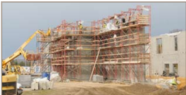
Construction crews work on the AT/MOB facility. Photo by Tom Michele
