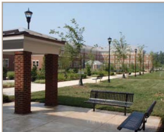
Warrior in Transition barracks at Fort Belvoir, Va., completed during FY 2011 can house 288 Soldiers. Photo by Edward Emden
