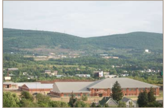
The Scranton Armed Forces Reserve Center, nestled in the hills of Pennsylvania, is built atop a former coal mine, a site that presented issues to be addressed. Photo by Michael Stewart
