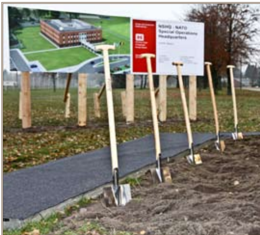
Shovels await the start of a groundbreaking ceremony Nov. 30, 2010, in Mons, Belgium, to mark the construction start for the $20 million NATO Special Operations Headquarters. Photo by Carol E. Davis
