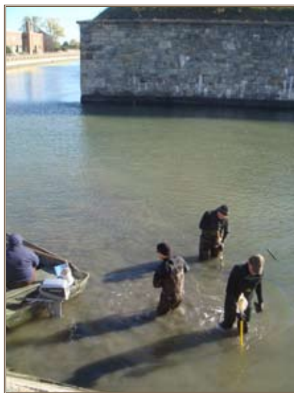
Contractors sweep the Fort Monroe moat for munitions. Photo courtesy of Science Application International Corporation
