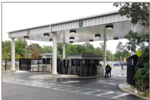
A gate at the Army National Guard Readiness Center in Arlington, Va., is an example of full life-cycle support from the Access Control Point Program.
