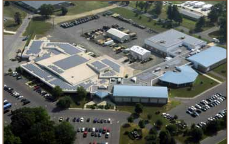
Solar panels cover about 71,000 square feet of roof surface at the New Jersey Guard's Battle Lab. Photo by Master Sgt. Mark C. Olsen, U.S. Air Force
