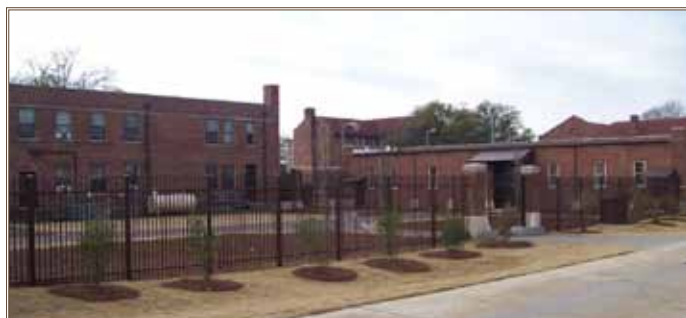
The twin buildings that underwent renovation at Fort Bragg form two sides of a courtyard. Photo by John Kahler, Directorate of Public Works, Fort Bragg
