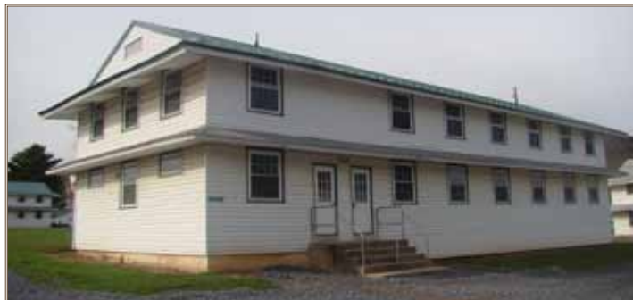
The newly restored Area 13 at Fort Indiantown Gap features historic brick structures and 21 World War II-era wooden barracks. Photos courtesy of Pennsylvania Army National Guard
