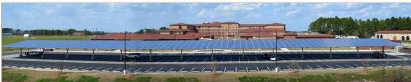
A PV array shades the Fort Bragg Warriors in Transition complex parking area. Photo by Paul Hora
