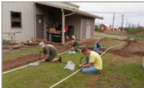
Boy Scouts install the irrigation system that will be supplied by rainwater collected from the OANRP building's roof. Photo by Hayley Diamond
