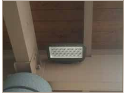
Fort Wainwright will test outdoor LED fixtures over the winter to see how well they perform in Alaska's extreme conditions. Photo by Sean Bogren
