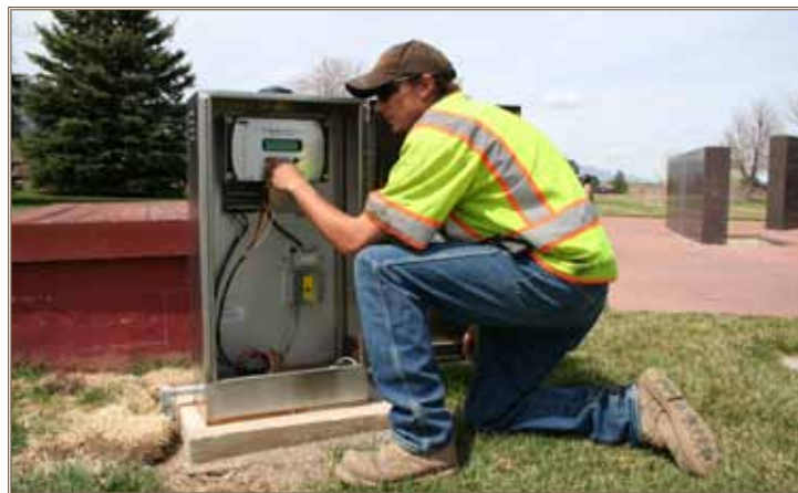
John Bishop, Fort Carson Support Services irrigation repair technician, monitors one of the evapotranspiration-system clocks. Photo by Susan C. Galentine
