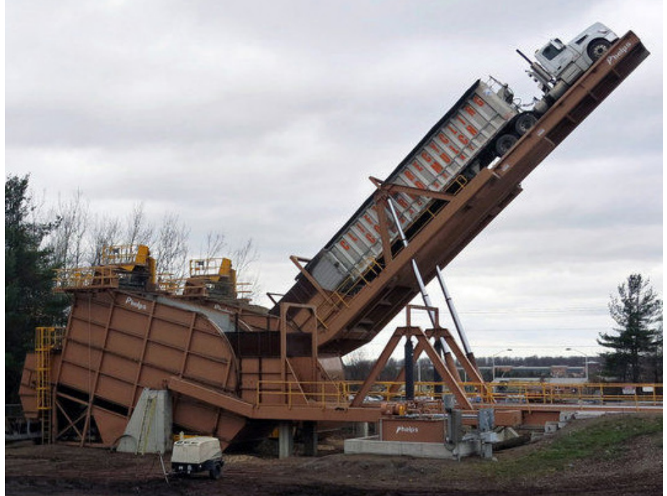
Wood chip truck unloading operation, Black River Power Plant, Fort Drum
