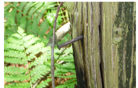
Machine-cut nail embedded in fence post at Fort Bragg (ERDC-CERL).
