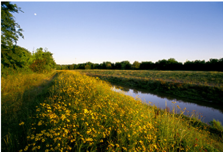
Work will start on the Greens Bayou Flood Damage Reduction Project this year.
