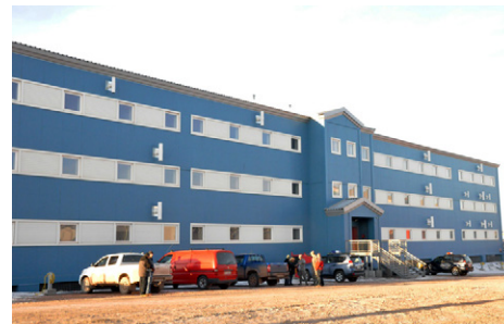
The 54 person dormitory under construction. (Castagna)
