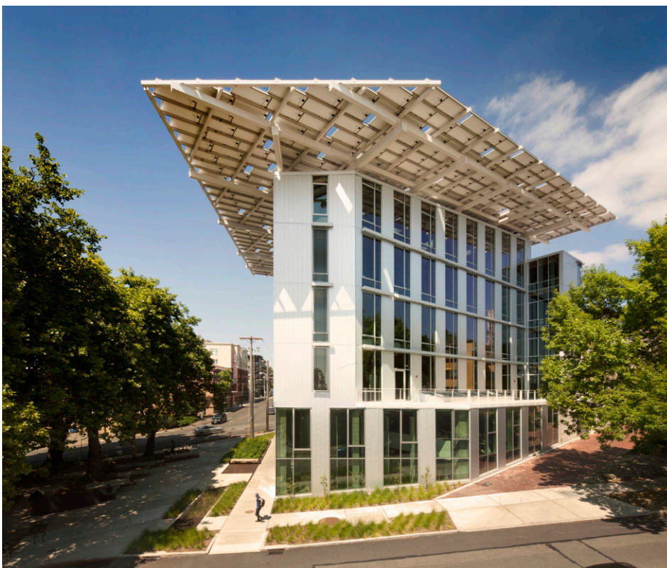
General view of Bullitt Center looking from across East Pike Street - Note roof profile extending over sidewalk to allow an increased number of photovoltaic panels to be installed on the roof.
