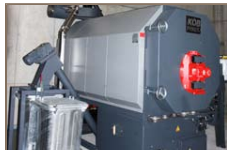
A biomass heating system is among the energy-efficient features in the new Logistics Distribution Center in Germersheim, Germany. Photo by Jennifer H. Aldridge
