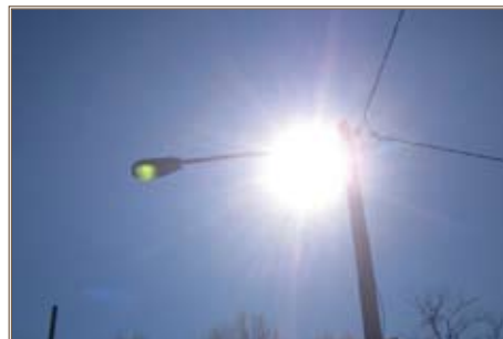
Unnecessary lighting such as this exterior lights on during daytime hours can be corrected for little of no cost.
