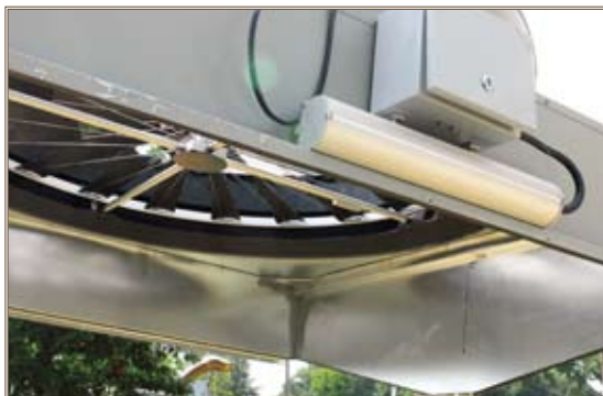
This wind turbine is designed to capture updraft from air-conditioning units and convert it into reusable energy. Photo by Vince Little
