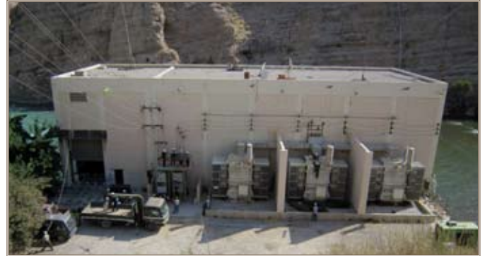
Kajaki Dam power house, built by the United States in the 1970s, provides power to residents of Helmand and Kandahar provinces. Photo by Chief Warrant Officer 5 Thomas B. Black
