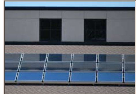
The PV panels on a Fort Bragg dining facility feed a solar domestic hot water system. Photo by Jonelle Thompson
