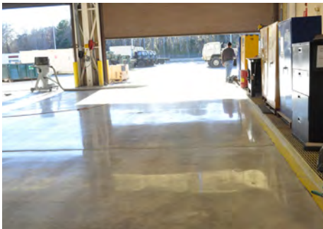
The new floor sealant is performing well after one year. (ERDC)
