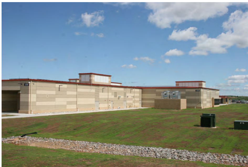
A look at the Reception Complex where the photovoltaic panels are in place on the roof. They are just visible on the roof above the two HVAC units. (B. Purdum)
