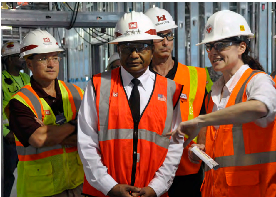
Fort Worth District chief of Engineering and Construction, Brian Giacomozzi and Fort Hood's director of Public Works, Brian Dosa look on as Erica Trovinfal, the Health Facilities Planning Agency project coordinator, briefs USACE Commander, Lt. Gen. Thomas Bostick, during an April tour of the hospital replacement project site in Fort Hood, Texas.
