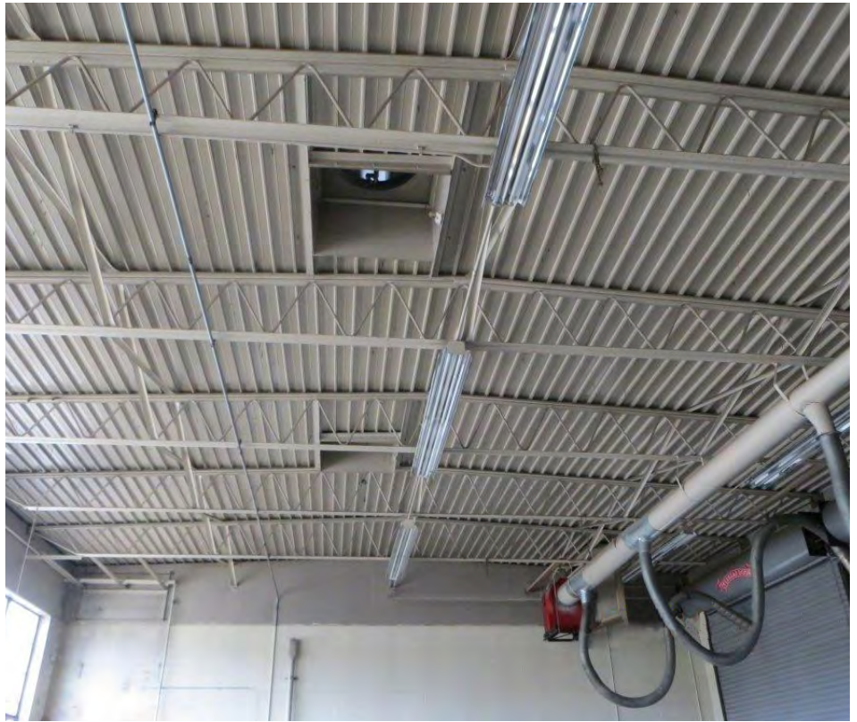
Insulation will be added to the ceiling
