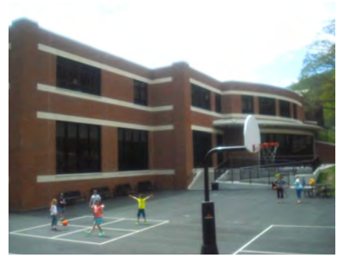
Completed West Point Middle School New Addition. (USACE, New York District)
