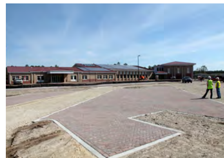
The new Murray Elementary School includes 456 solar photovoltaic panels and 10 solar water heating panels on the roof. These panels will augment the facility’s total electrical usage and heat about 40 percent of the building’s hot water. (G. Jumara)
