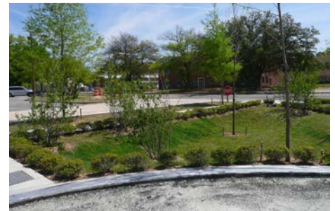
This vegetated swale sited in the cantonment at Fort Bragg, N.C., is an example of a LID feature which is compatible with a historic district. (Photo courtesy of U.S. Army)
