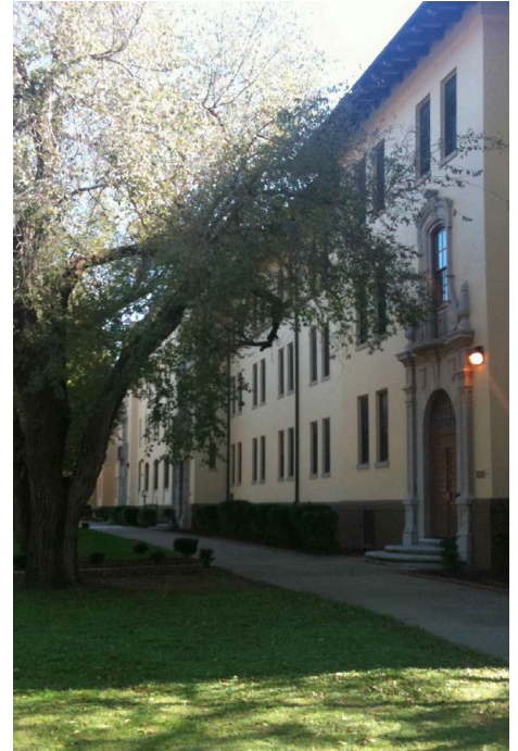
Many older buildings, including this one at Fort Sill, were designed with narrow wings and numerous windows so that all occupants could have access to natural light and cooling breezes.
