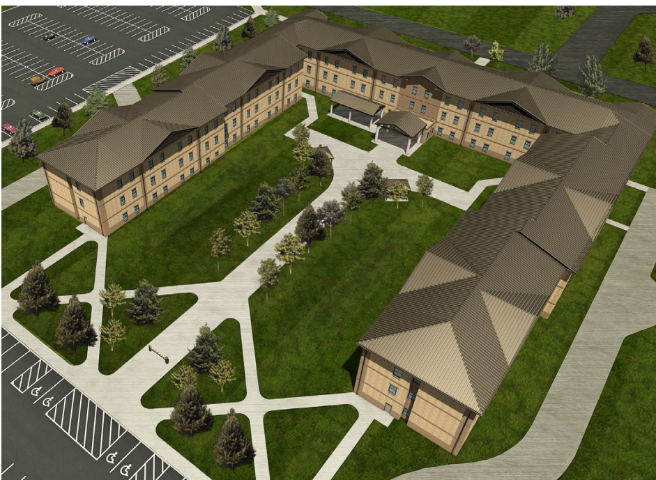
A rendering of the new three-story HHB barracks at Fort Campbell that will house 296 Soldiers.
