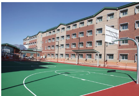
These barracks, located in Fort Carson, Colo., have been constructed in close proximity to Butts Army Airfield. (Weddington, USACE)
