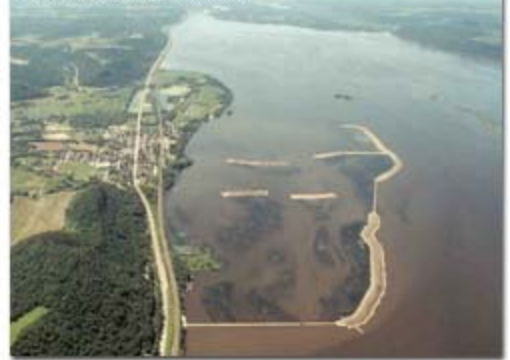
Islands and rock sills constructed in pool 8, Stoddard, Wisconsin.
