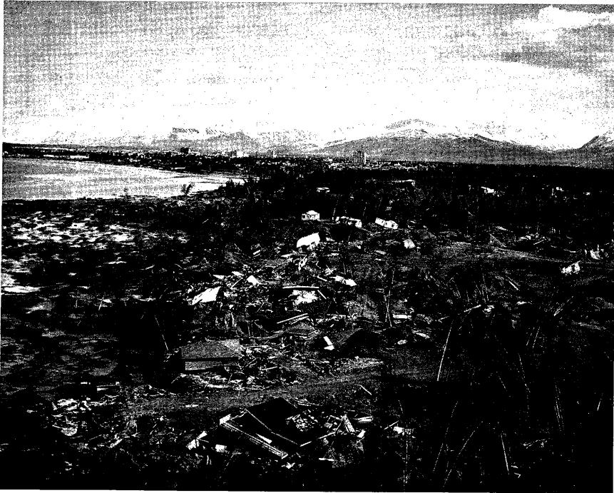
Earthquake damage, Turnagain residential area, Anchorage.
