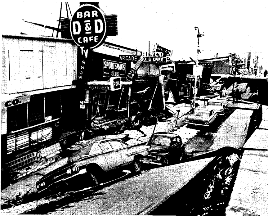
Earthquake damage, central business district, Anchorage.
