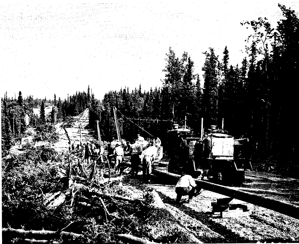
Construction of the Haines-Fairbanks military pipeline, 1954.
