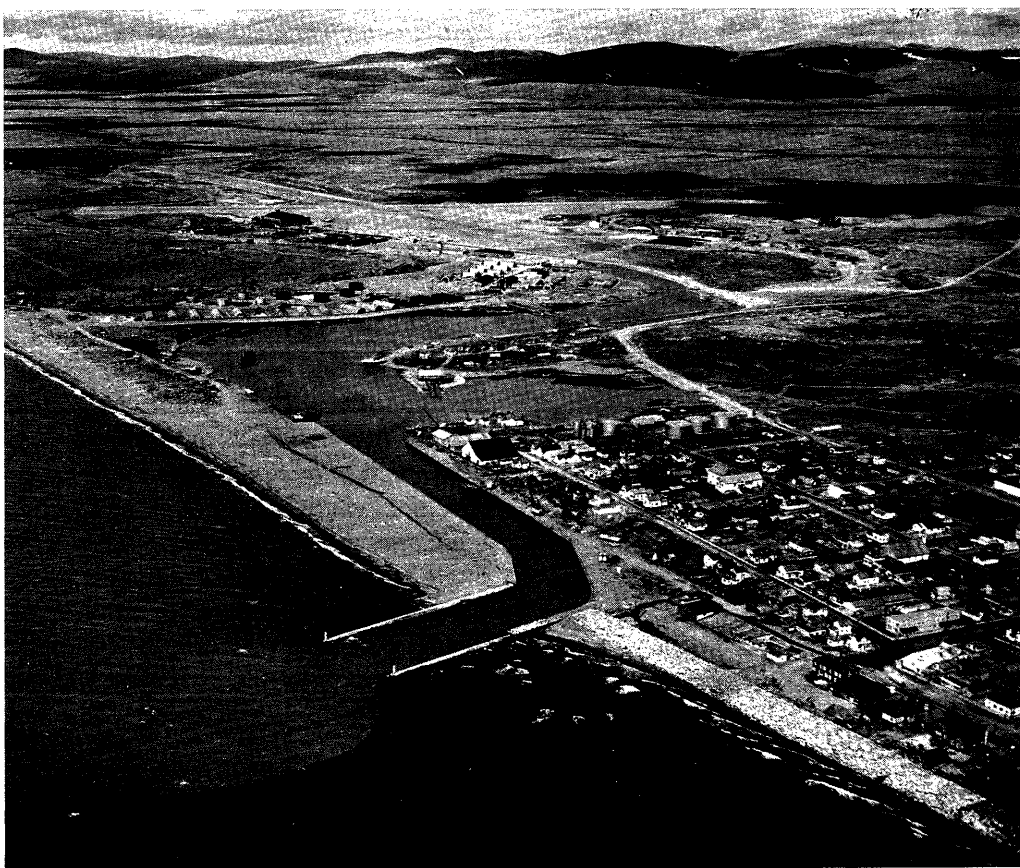
Jetties, channel, and turning basin at Nome. Sea wall is at right of harbor entrance.
