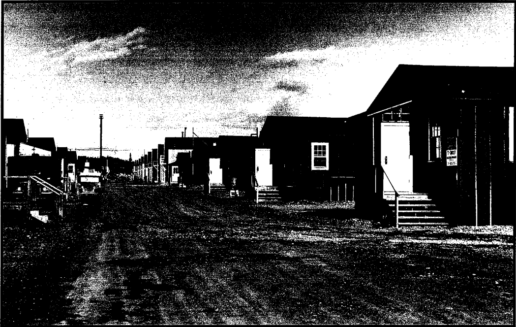
Street in construction camp area.
