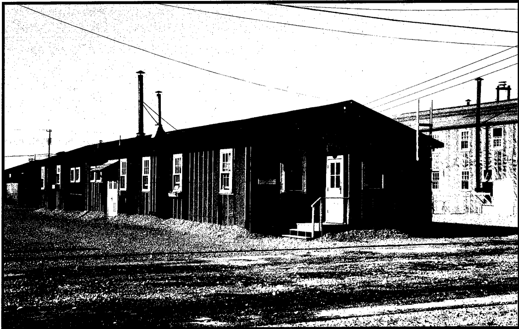
Typical barracks building.
