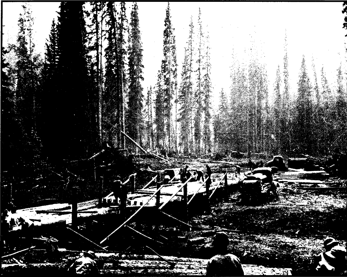
Trestle bridge under construction on the Alaska Highway.
