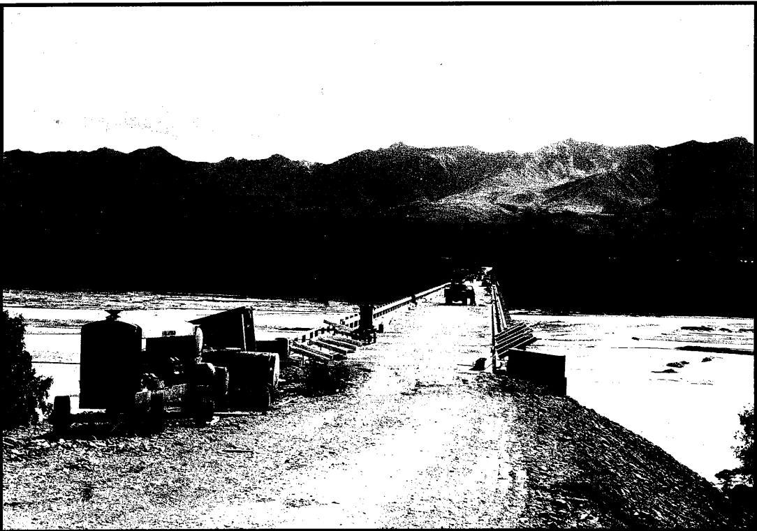
Looking south across the Northway Bridge, 1944.
