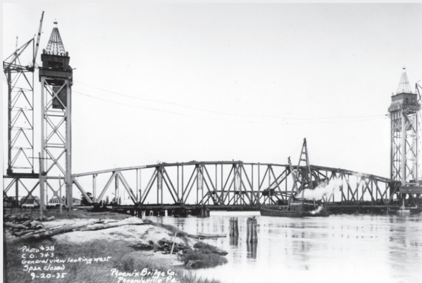
Construction of the Cape Cod Canal Railroad bridge located in Bourne, Mass., 1935.
