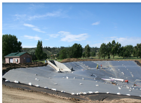
Fort Carson's golf course holding pond is undergoing expansion to double its capacity to carry 30 million gallons of water to accommodate a reclaimed water project for irrigation on post.
