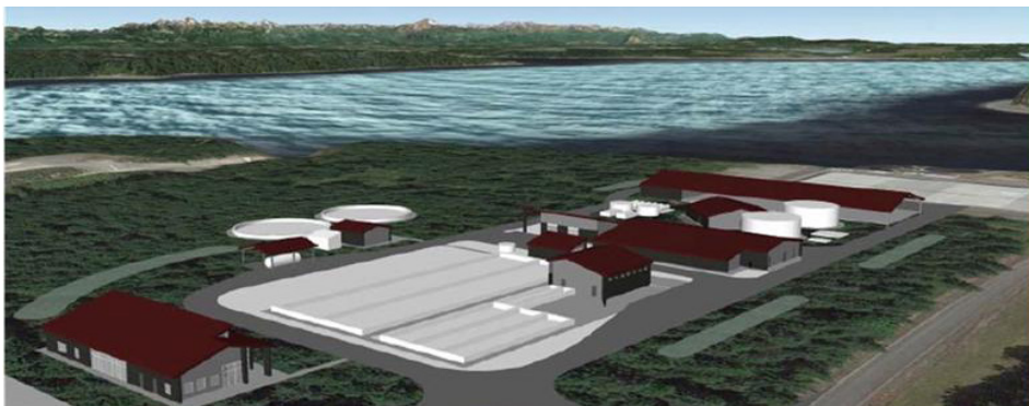
Wastewater Treatment Plant flyover view with the Puget Sound in the background. (CDM-Smith)
