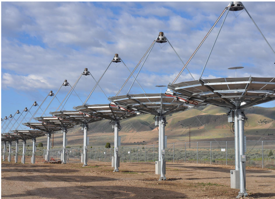
429 solar dishes at Toole Army Depot are expected to provide 1.5 megawatts of electricity, approximately 30 percent of the depot's annual electric energy need. (Anderson, Toole Army Depot)
