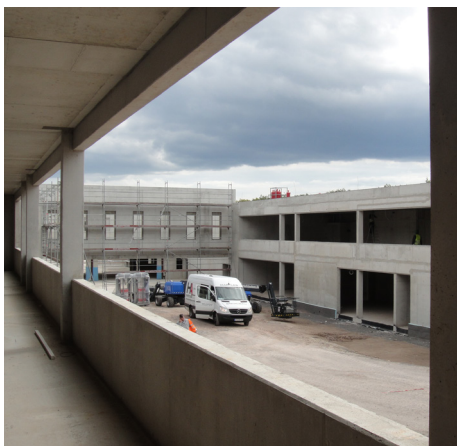
Several large bays for windows to get maximum sunlight illumination
