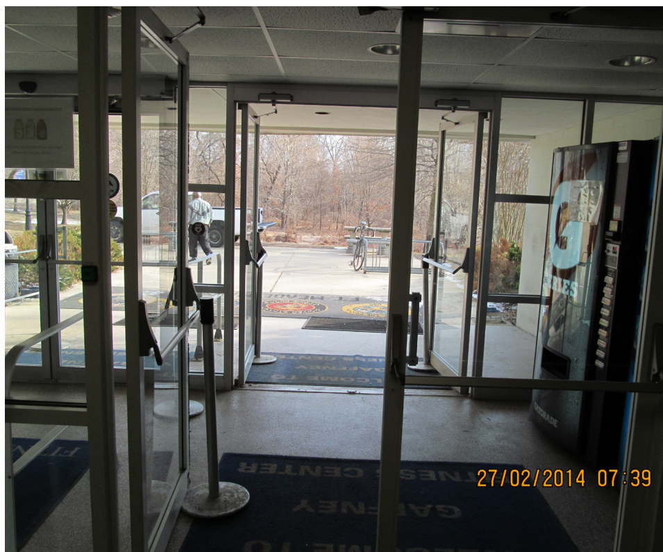
A common example of energy waste found during an assessment is inner and outer vestibule doors propped open.
