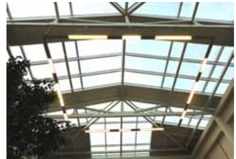
A typical energy conservation measure using skylights to provide adequate lighting during daytime
