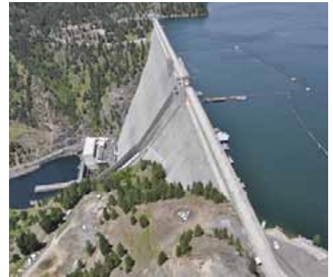
400 MW capacity Dworshak Dam, located in Idaho.
