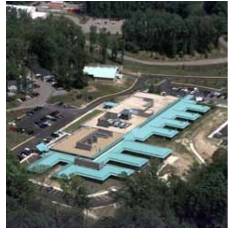
This aerial shot of ITL at Vicksburg, Miss., shows some of the massive chiller equipment required to cool the supercomputers inside the facility. Photo courtesy of ERDC
