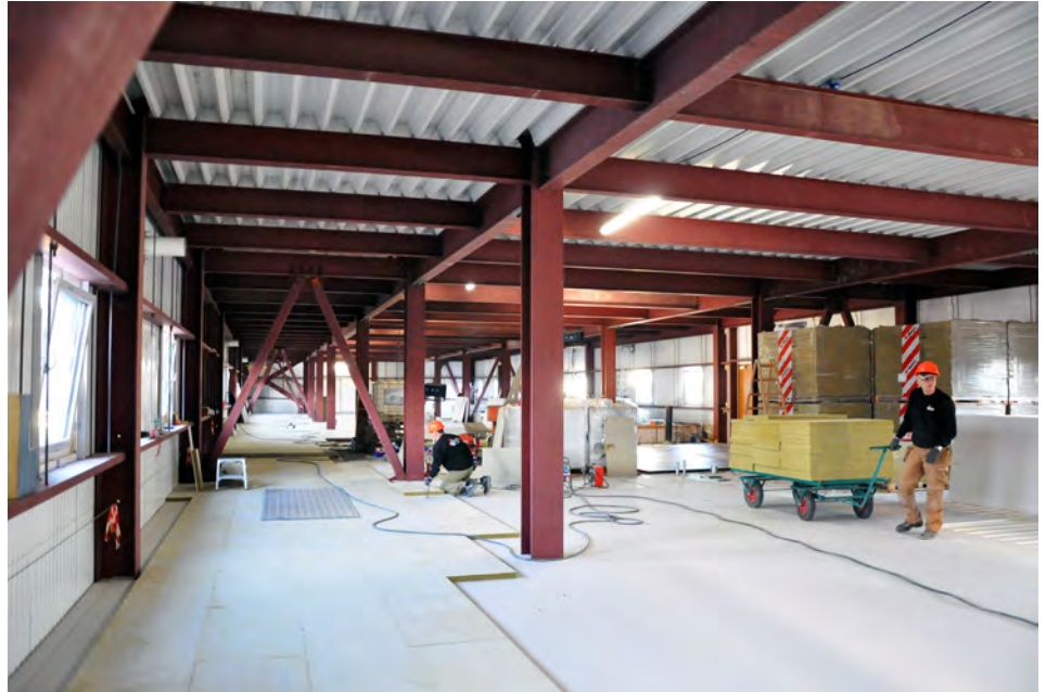
Contractors working inside one of the dormitories. Photo by JoAnne Castagna
