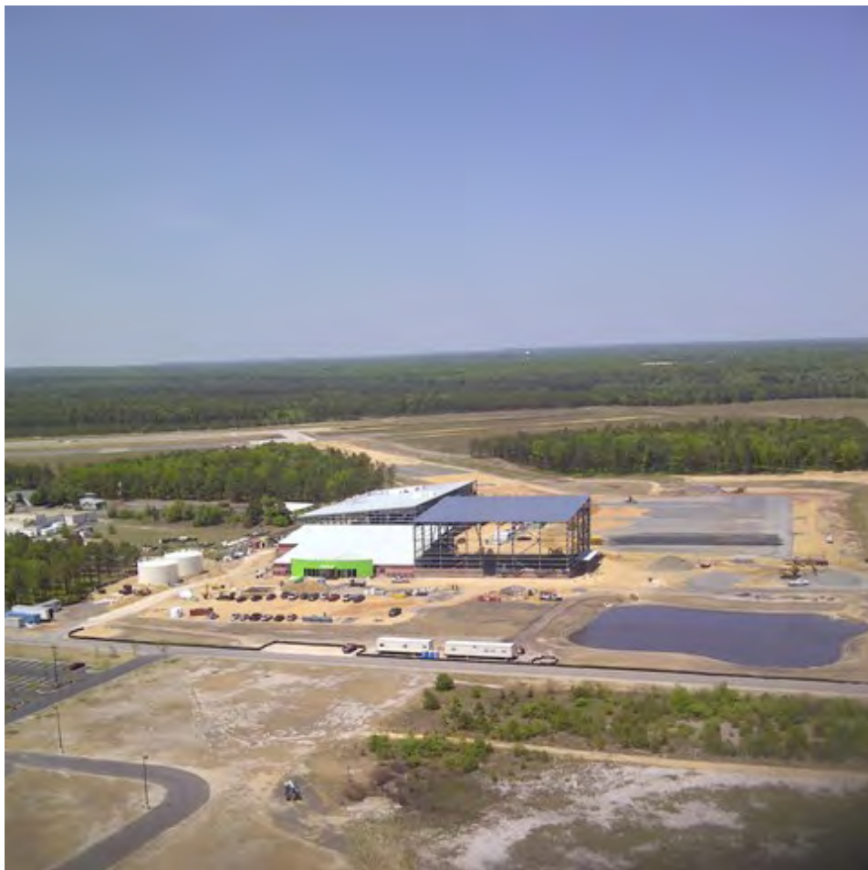
Aerial of complex under construction in May 2015. Photo by RC Smith.
