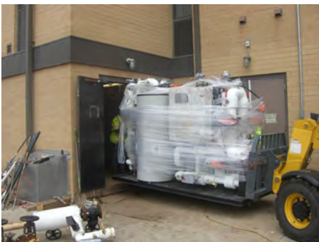
Mechanical equipment room skids are compact, energy-efficient systems that can be quickly installed into a facility mechanical room as one unit, minimizing utility down time in the buildings. Photo by Bruce Faul
