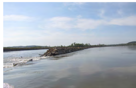
Revetment notch on Missouri River. Photo by Dereck Wansing
