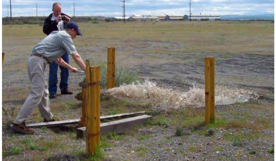
Personnel at Umatilla performing annual flushing. Courtesy photo
