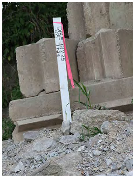
Stakes inform workers of dike numbers and locations. Photo by Trisha Dorsey
