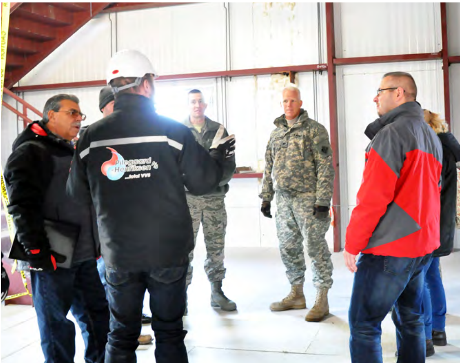
Engineering team discussing one of the dorm construction projects. Photo by JoAnne Castagna
