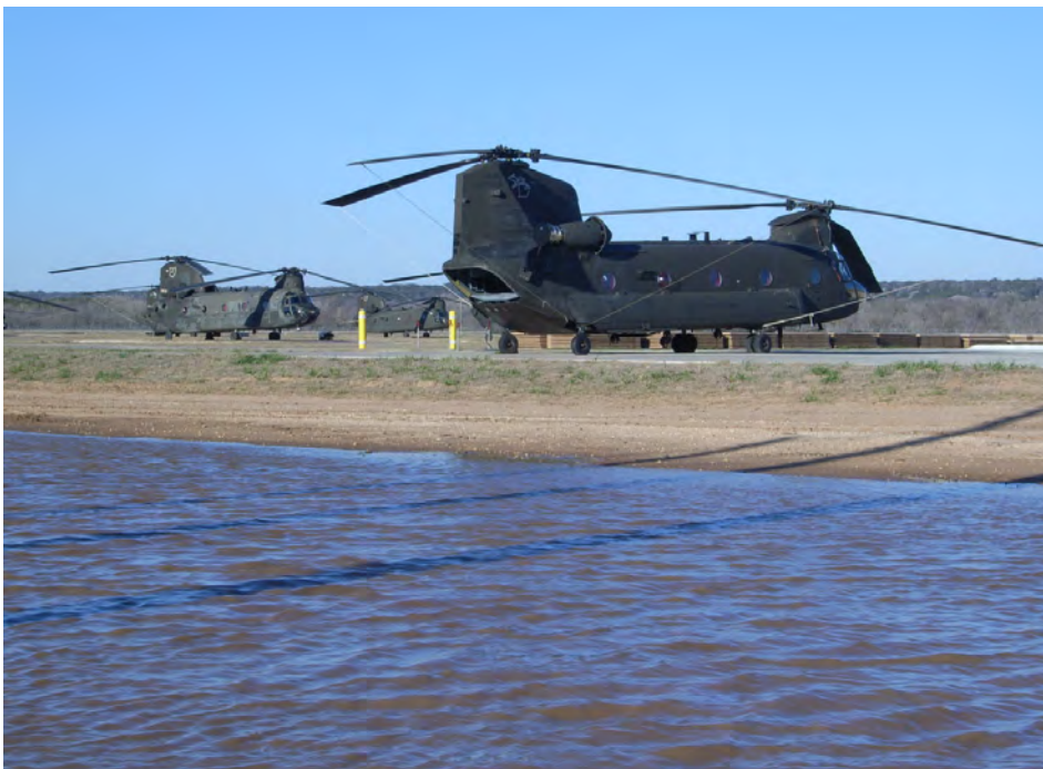
Ponding near Longhorn Airfield could create potential damage to important infrastructure and military equipment. A plan to improve stormwater was needed to reduce damages from storm events. Courtesy photo
