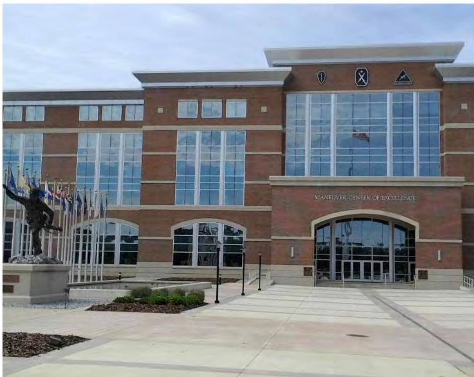
The newly renovated McGinnis Wickam Hall (headquarters for the Maneuver Center of Excellence), Fort Benning, Georgia. Photo by Geoff Ray
