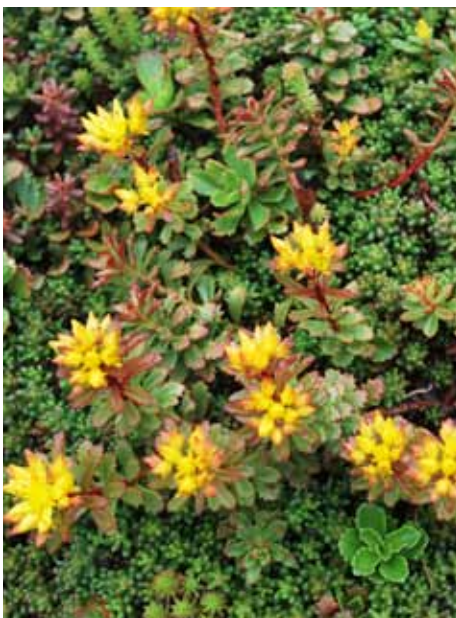
LiveRoof1: The first vegetated roof at Fort Bragg features over 500,000 evergreen and deciduous sedum plants designed to manage storm water, reduce the urban heat island effect and conserve energy. Photo by Jonelle Kimbrough.
