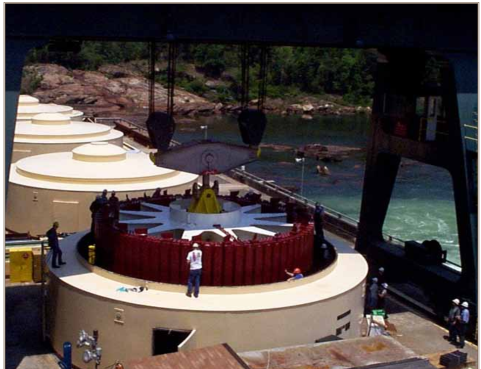
Hartwell Dam powerhouse generator repairs. Photo by Savannah District
