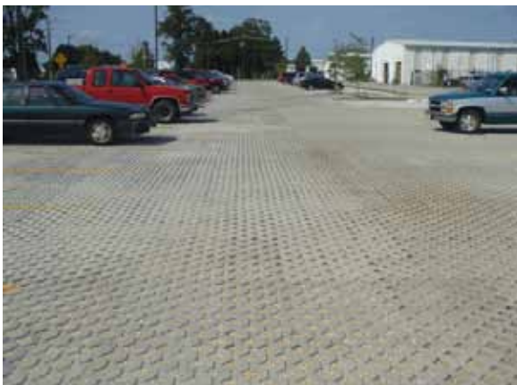
Permeable Pavers at Fort Lee, Virginia
