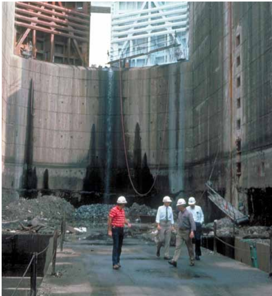
Wilson Lock dewatering inspections & repairs. Photo by Nashville District
