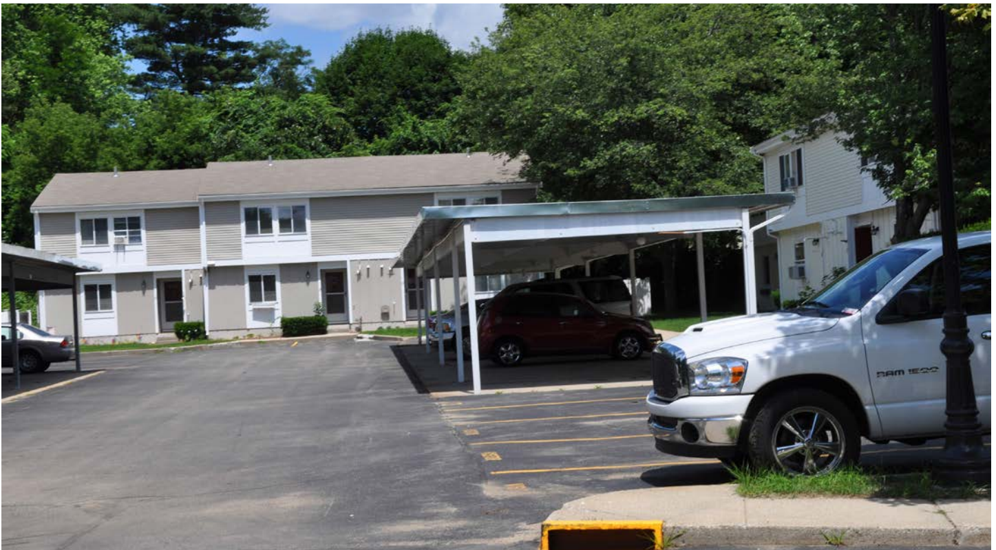
The U.S. Army Garrison Natick plans to replace family housing on Heritage Lane built in 1973 with new townhomes. (U.S. Army photo)
