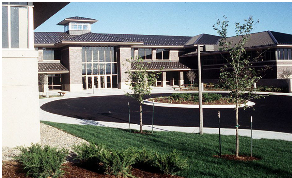
Rushmore Center is a consolidated administrative building at Ellsworth Air Force Base, South Dakota, with 50 foot-wide wings that allow most occupants to access great views and natural light. The Omaha District of the U.S. Army Corps of Engineers served as the design agent for this award-winning project. (Image courtesy of Mark L. Gillem)
