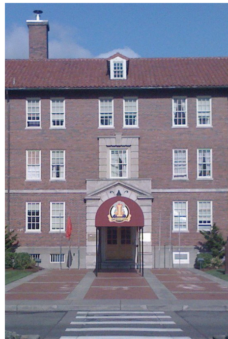
The historic I Corps headquarters at Joint Base Lewis-McChord, Washington, is an excellent example of a resilient building in a compact, walkable district. It uses durable materials, narrow wings, and high ceilings to improve energy-efficiency and create a desirable place to work and is within walking distance of other administrative buildings, family housing, and the installation's retail center. (U.S. Army photo)
