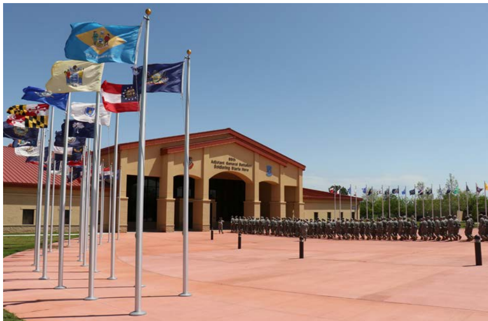
The Reception Battalion Complex at Fort Sill, Oklahoma, is a 93,000 square foot facility that includes medical and dental screening facilities, a uniform and equipment issue warehouse, barbershop and personnel processing offices. More than 20,000 men and women starting their Army careers will pass through the complex annually. (Photo by Ed Johnson)
