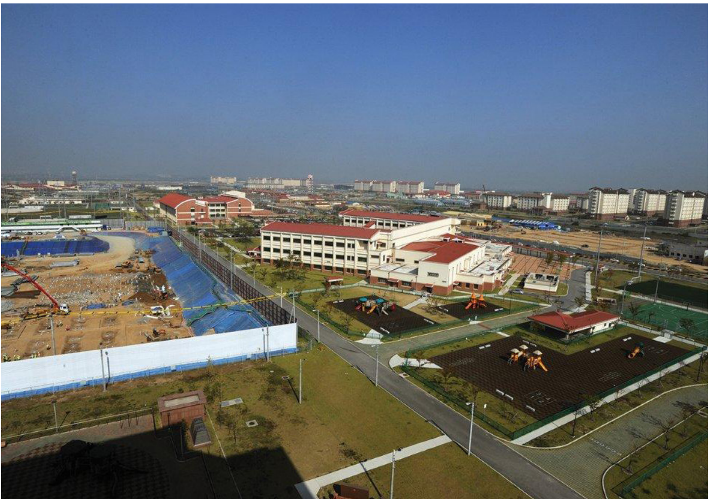
The new Camp Humphreys as seen from one of the recently built Family Housing Towers. New family housing is being built next door (left of photo), while schools, barracks and support facilities are all within walking distance of each other. (Photo by Bob McElroy)
