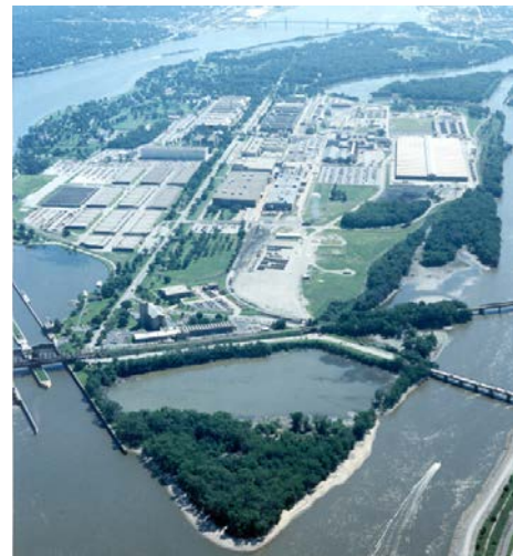
U.S. Army Garrison Rock Island Arsenal is one example of an atypical Army garrison. Weapons are crafted at the Illinois site, but it also provides for administrative space such as an office complex. (Photo courtesy of Woolpert)
