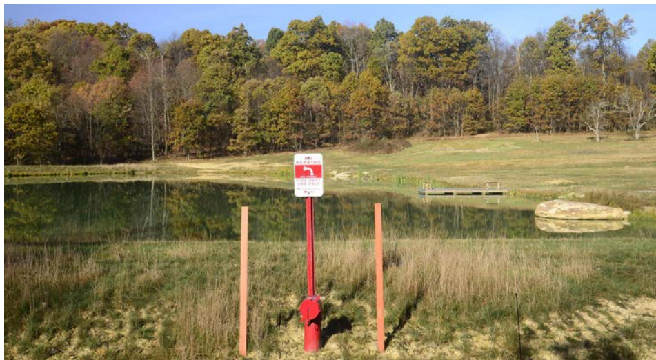
The completed pond project serves as a fire suppression source for the range and habitat enhancement for area wildlife. Recreation fishing at the pond also is planned. (U.S. Army Photo)
