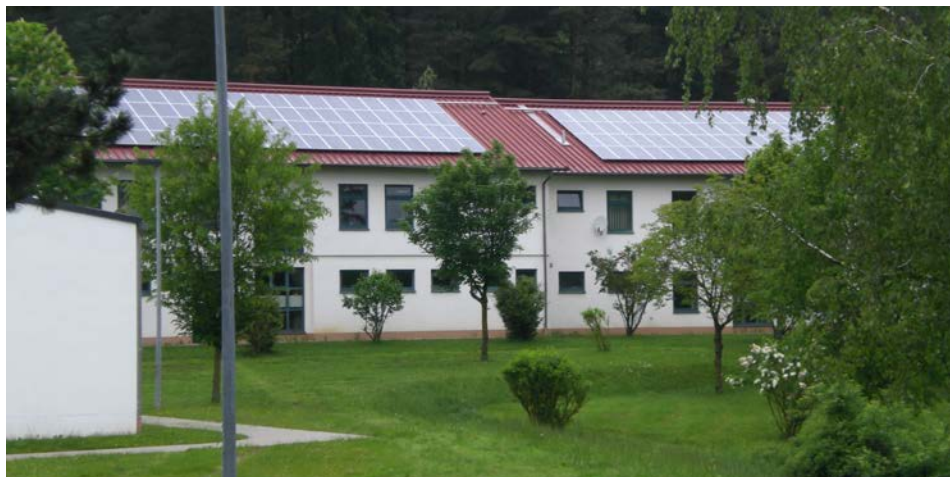
A roof-mounted photovoltaic system provides U.S. Army Garrison Bavaria housing electricity (U.S. Army Photo)
