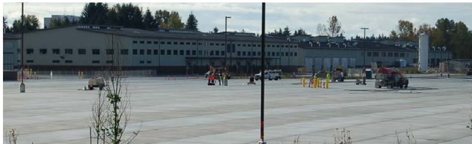
The I-5 pump and treat system at Joint Base Lewis-McChord provides heating for two tactical equipment maintenance facilities, annually saving approximately $50,000 in energy costs. (Photo by Tom Lynott)
