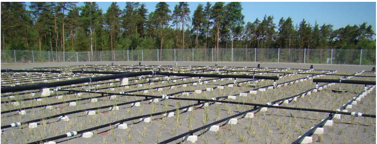
Treatment plant construction – shortly after completion
