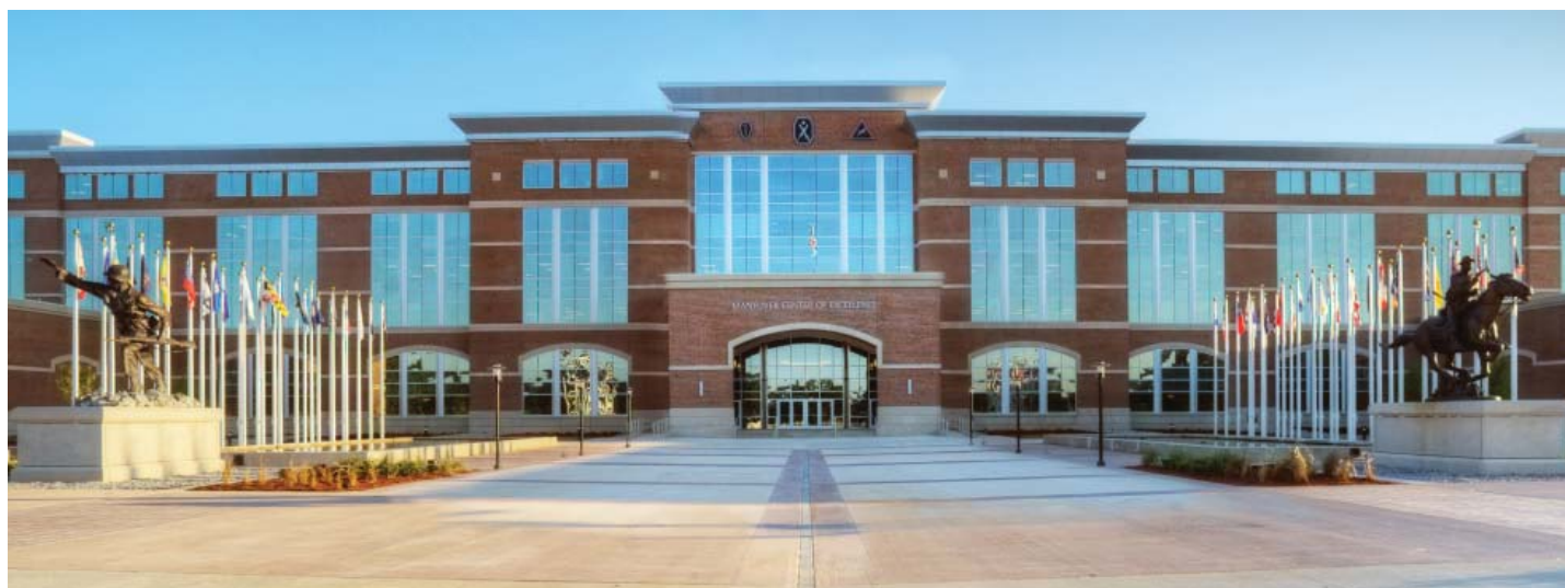
The U.S. Army Corps of Engineers Savannah District managed the $168 million renovation of the Maneuver Center of Excellence Headquarters at Fort Benning, Ga. The building achieved Leadership in Energy and Environmental Design Gold certification in December 2012. (Kristian Ogden)
