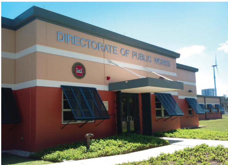
The New Directorate of Public Works front entrance façade. Note the South Gate Wind Turbine in the background one of two built under Fort Buchanan Energy Savings Performance Contract. (Francisco J. Méndez)
