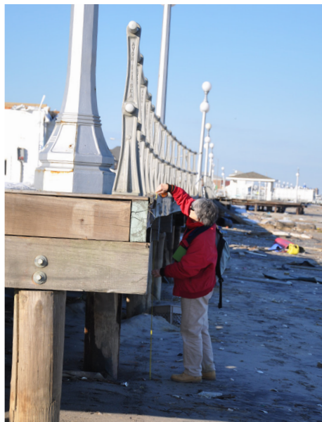
New York District Coastal Engineer Diane Rahoy assesses the Avon-by-the-Sea, N.J., coast November 9, 2012 after a nor'easter struck the area just days after Hurricane Sandy struck. (photo by Dan Desmet, New York District)
