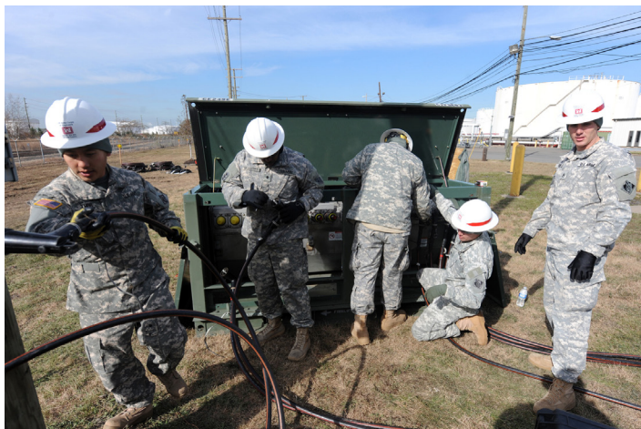
Soldiers from the 249th Engineer Battalion (Prime Power) install electrical generator equipment Nov. 6, 2012, at a Carteret, N.J., fuel depot that lost power during Hurricane Sandy. Power outages contributed to temporary gas shortages after the storm and getting fuel depots running was important to ending shortages. (DoD photo by EJ Hersom)
