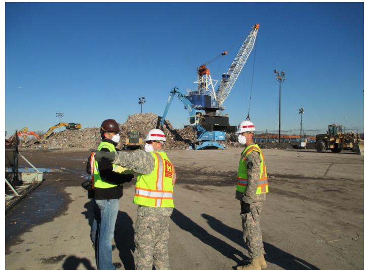
Army Corps personnel oversee debris operations at Fresh Kills Park in Staten Island, N.Y., where debris removed from private and public property is temporarily stored before being hauled to long-term sites. The Corps provided debris removal assistance after Hurricane Sandy as part of a FEMA mission assignment. (photo by Ron Fournier, Rock Island District)
