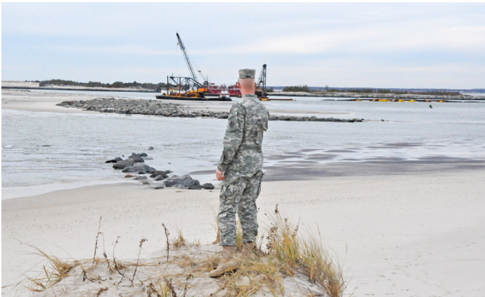
New York District Commander Col. Paul E. Owen stands on the edge of a dune and looks over a barrier island breach in Cupsogue County Park on Long Island Nov. 16, 2012, that was created by Hurricane Sandy. Crews are visible mobilizing to begin breach closure operations. (photo by Chris Gardner, New York District)
