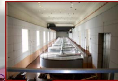
Bull Shoals Powerhouse Arkansas
