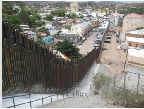
Nogales, Ariz., Border Fence Replacement
